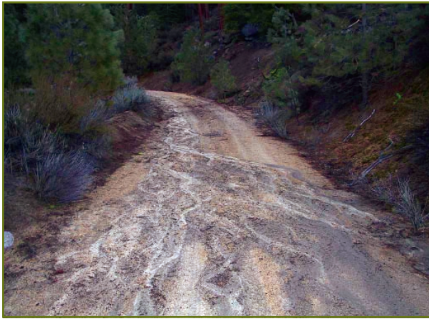
Erosion on dirt road.
