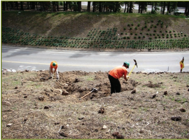
Loosening soil by hand using pick mattocks.
