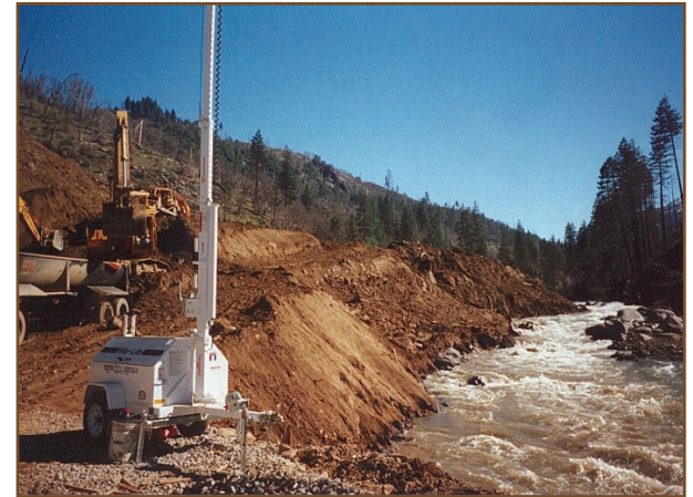
This photo of the American River shows a mass failure that temporarily blocked the river. This slide was believed to be the result of lack of vegetation from a previous fire, defoliation efforts, and water associated with a 100-year precipitation event (1997).
