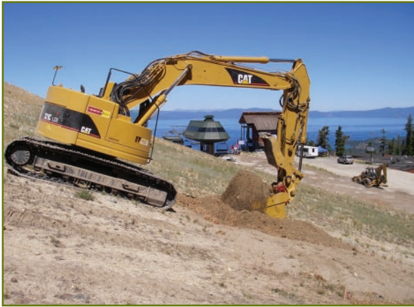
Constructing test plots on ski run at Heavenly Mountain Resort
