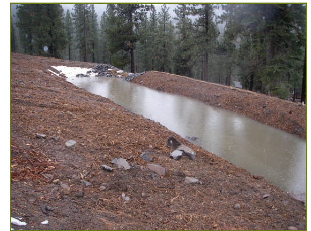
Settling basin near capacity during an early winter storm.
