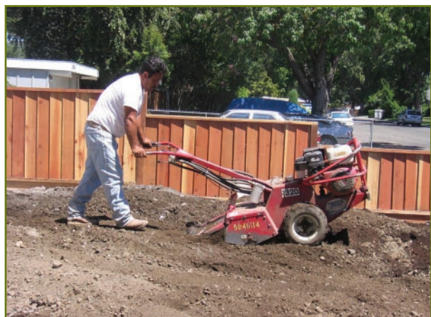
Loosening soil with hand-operated rototiller.
