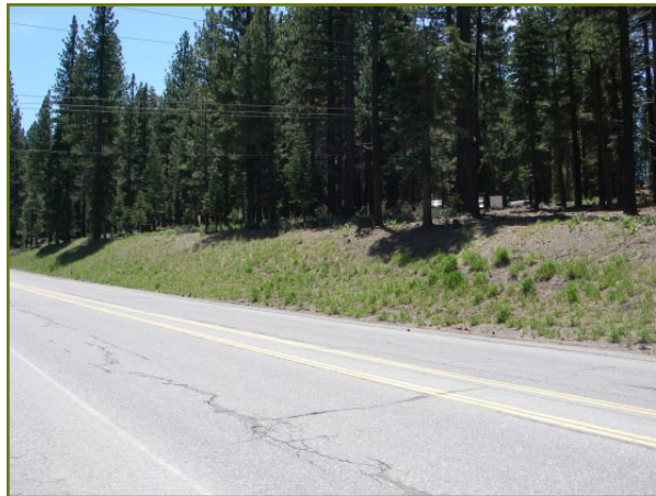
Highway 267 slope, three years after treatment.
