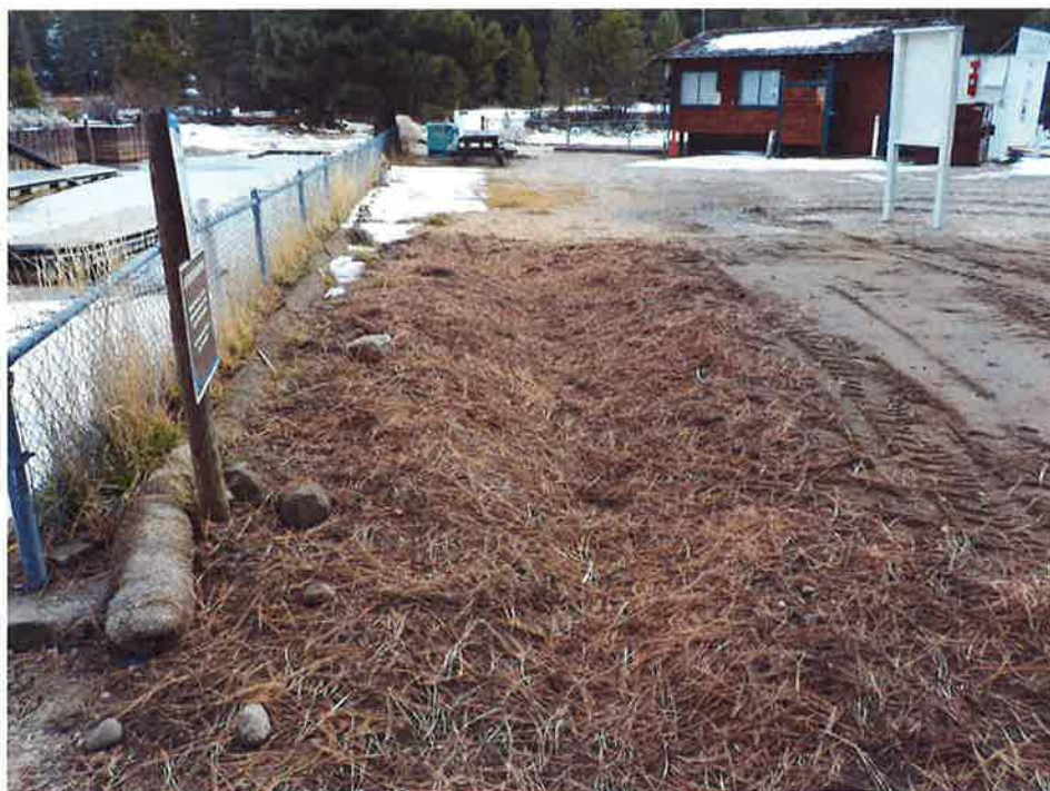
December 8, 2015. Swale looking south at STA EAST 1+50 following construction.
