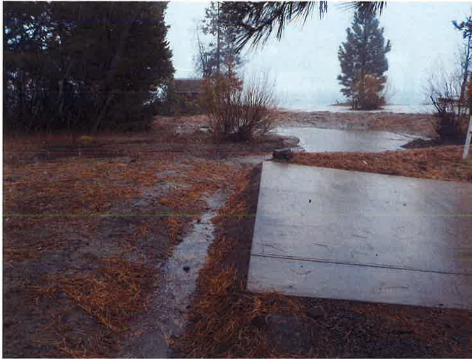
December 10, 2015. Swale and basin looking east at STA EAST 2+00 following precipitation.
