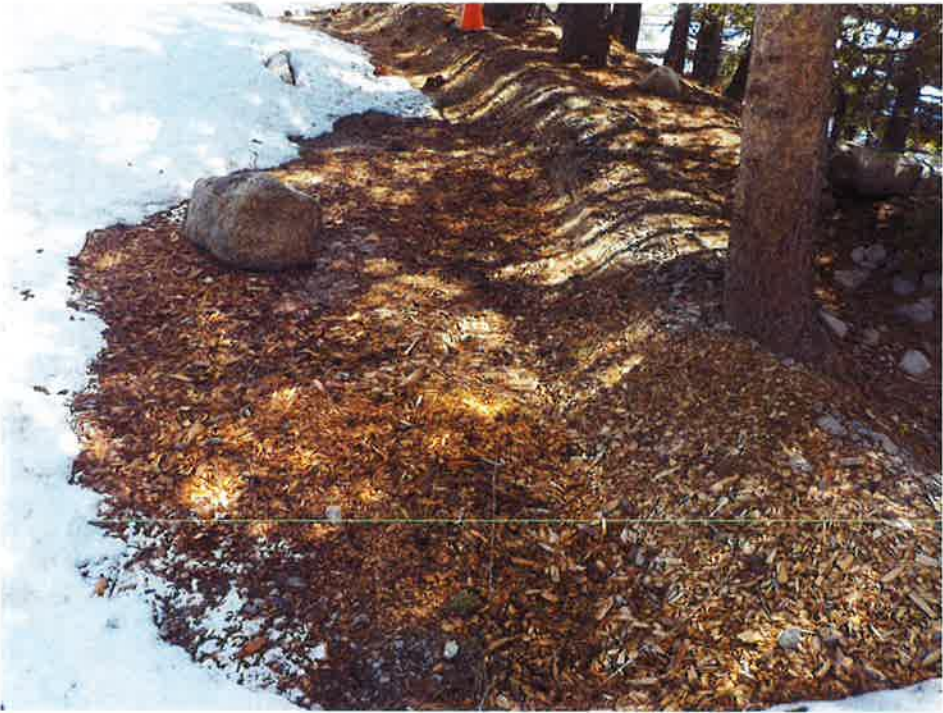
April 20, 2017. Swale and berm looking east at STA 0+00.
