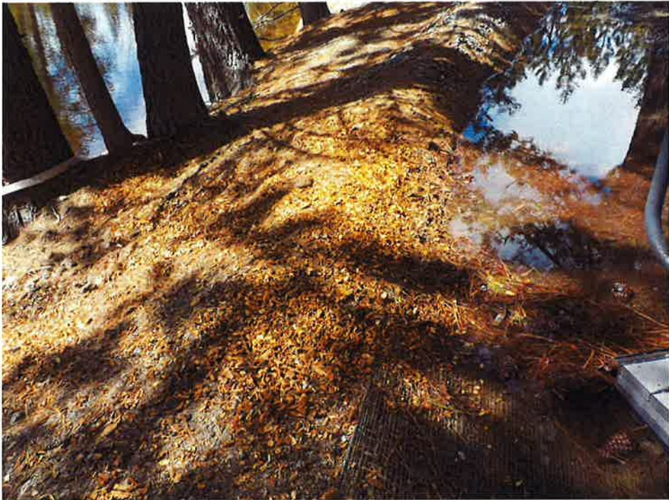
April 20, 2017. Repair of eroded berm at STA WEST 2+40 looking west.
