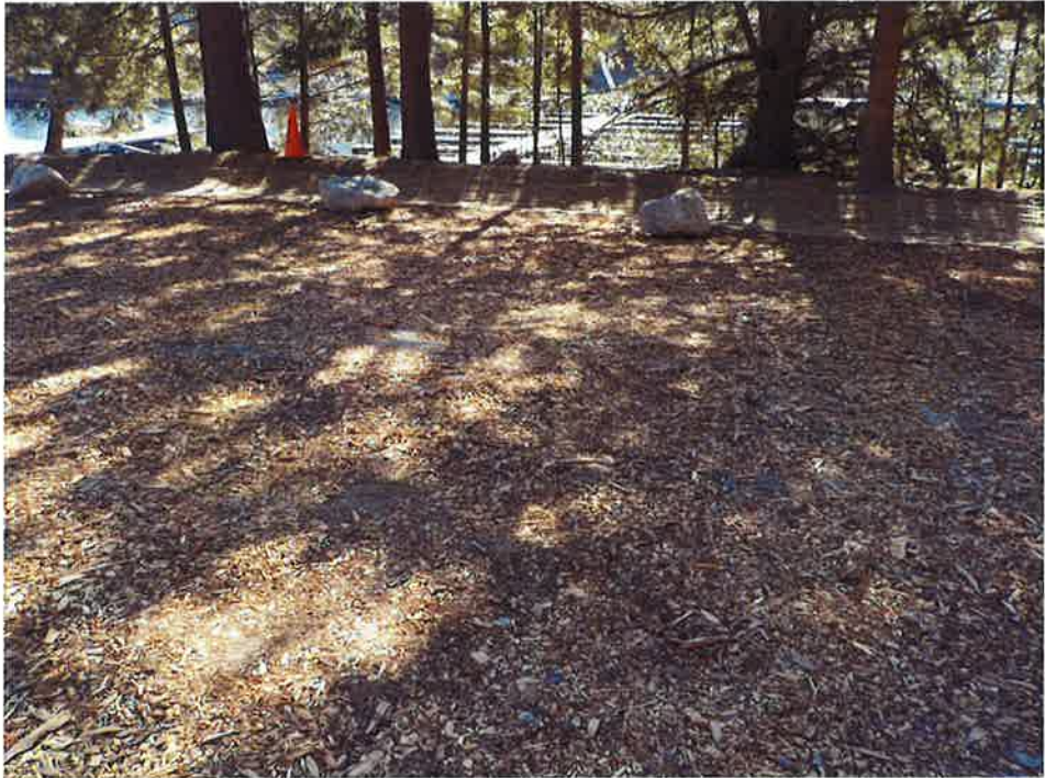
October 12, 2016. Swale and berm looking south at STA 0+00 following construction.
