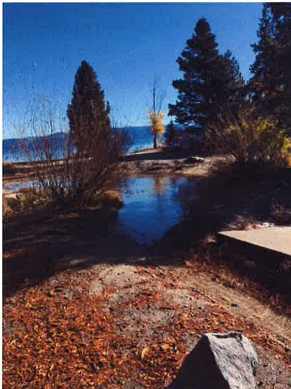
November 1, 2016. Basin, swale and berm at STA EAST 1+80 following precipitation.
