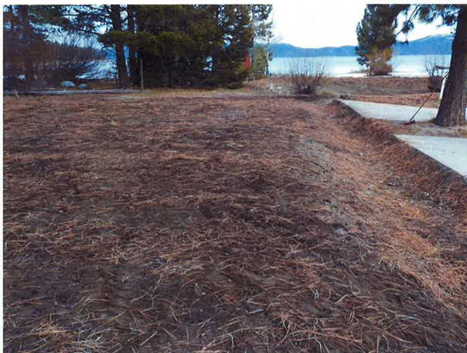
December 8, 2015. Swale looking east at STA EAST 1+50 following construction.
