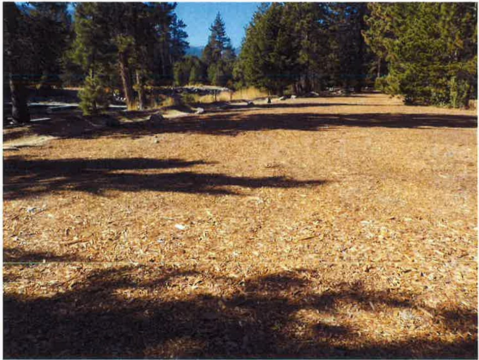
October 12, 2016. Day use parking area looking west at STA 0+00 following construction.
