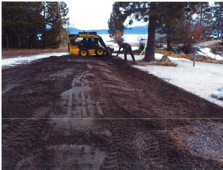
December 8, 2015. Swale construction looking east at STA EAST 1+50.
