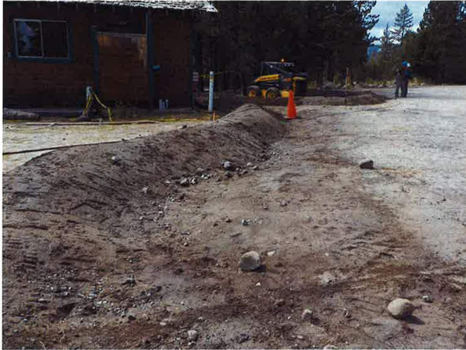
September 13, 2016. Swale and berm construction looking west at STA 0+00.
