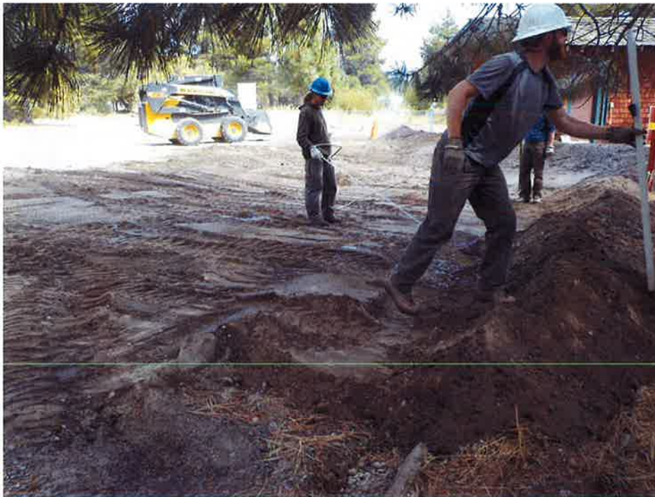
September 13, 2016. Basin and berm construction looking east at STA 0+00.
