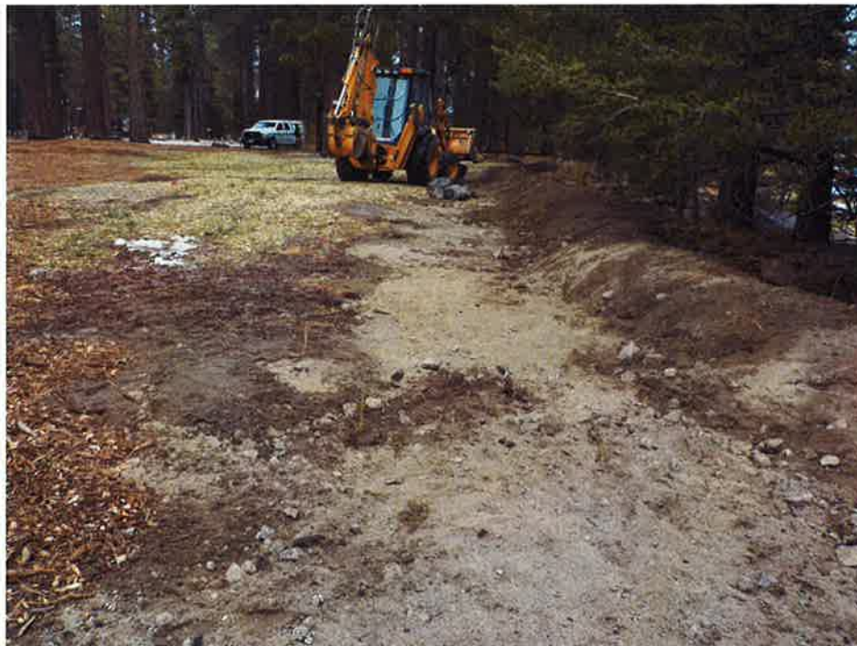
October 3, 2016. Swale and berm construction looking east at STA EAST 3+40.
