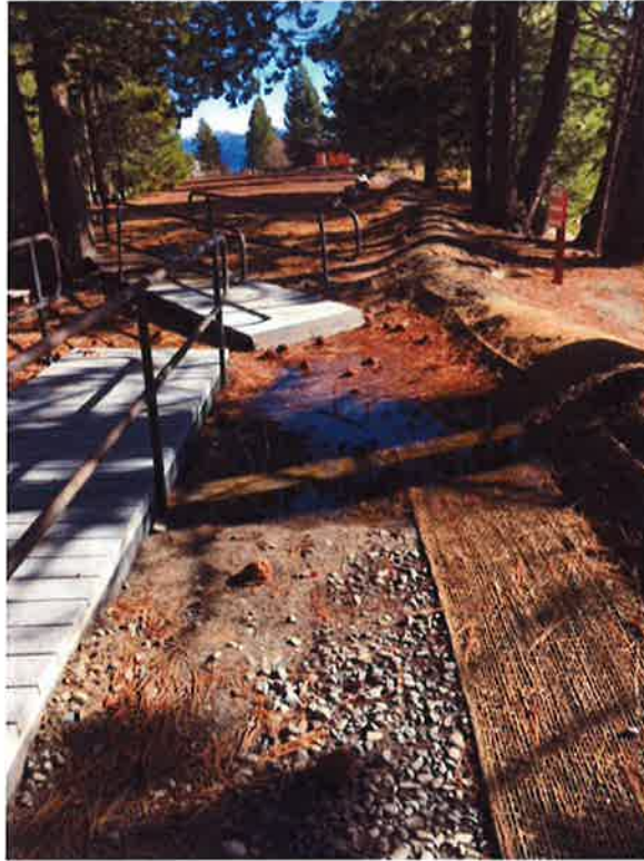
November 1, 2016. Swale and berm at STA WEST 2+40 following precipitation.
