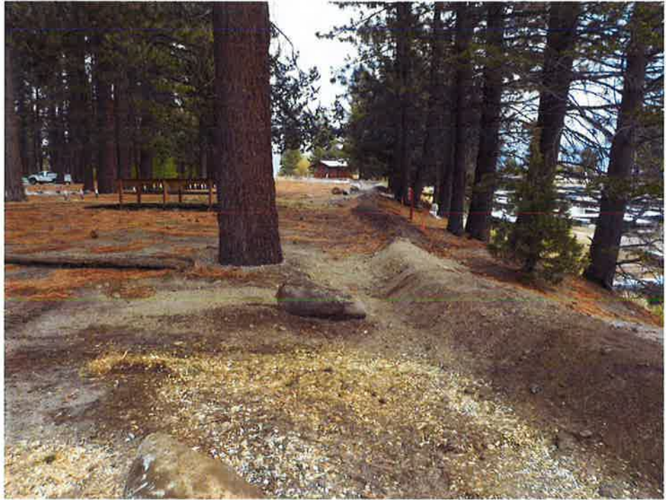
October 3, 2016. Swale and berm construction looking east at STA EAST 2+40.
