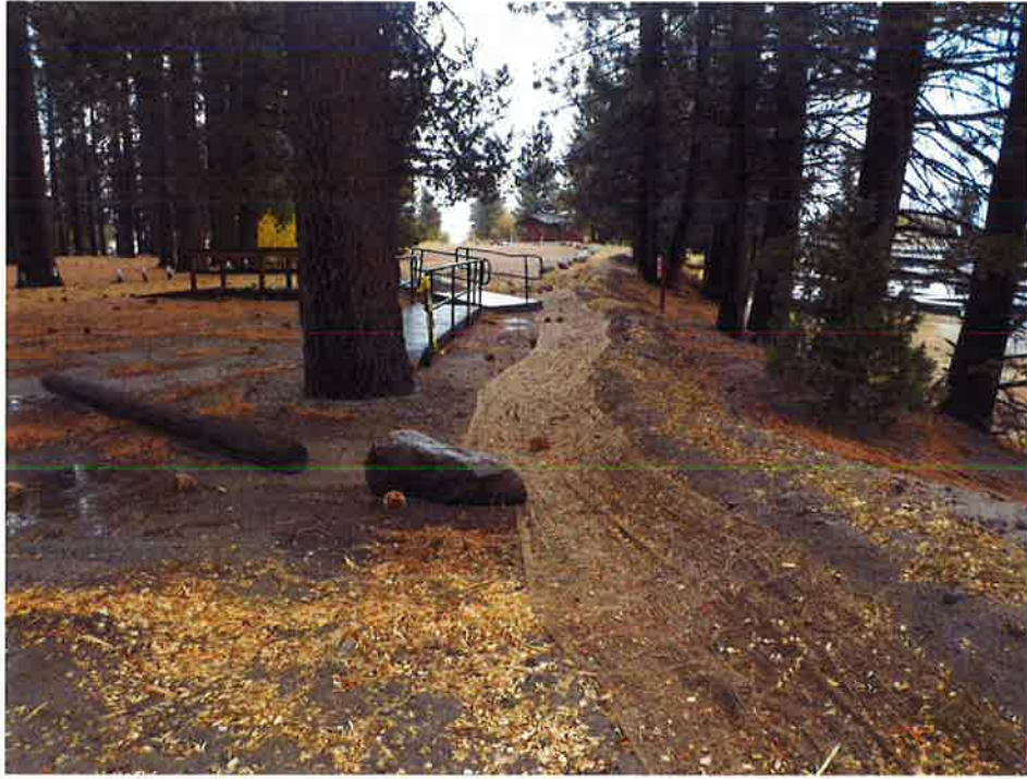
October 14, 2016. Swale and berm looking east at STA WEST 2+40 following precipitation.
