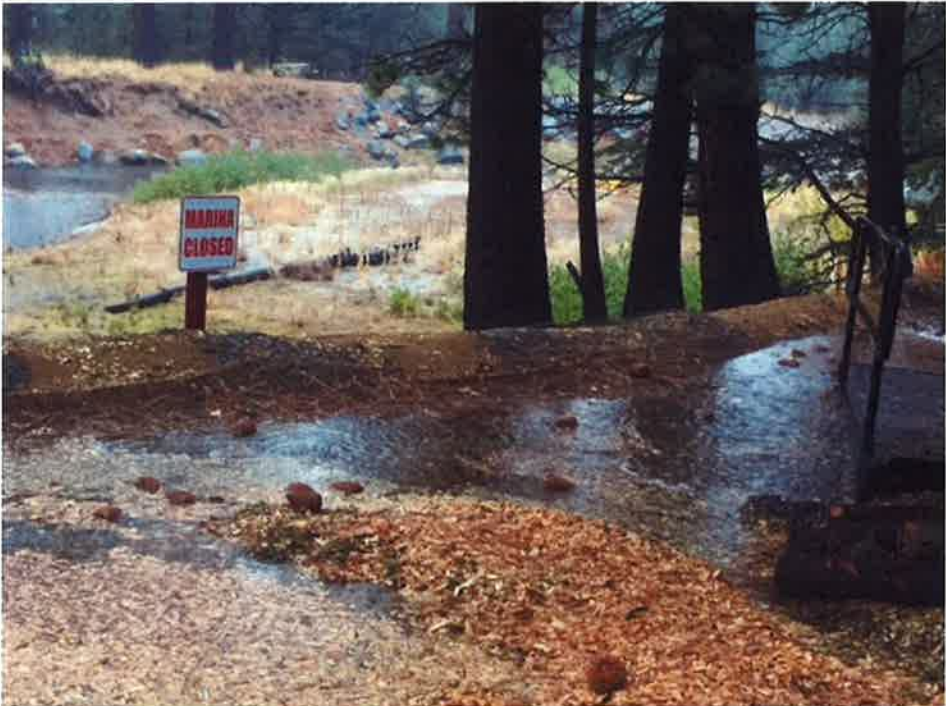
October 16, 2016. Swale and berm looking south at STA WEST 2+40 following precipitation.
