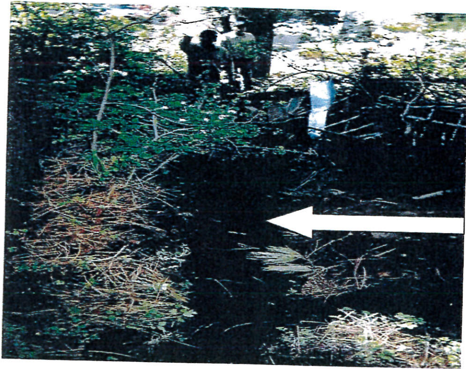
Photo 14. A new drainage ditch below West Reed Avenue that was being dug on May 29, 2006 to convey runoff to Donner Pass Road.
