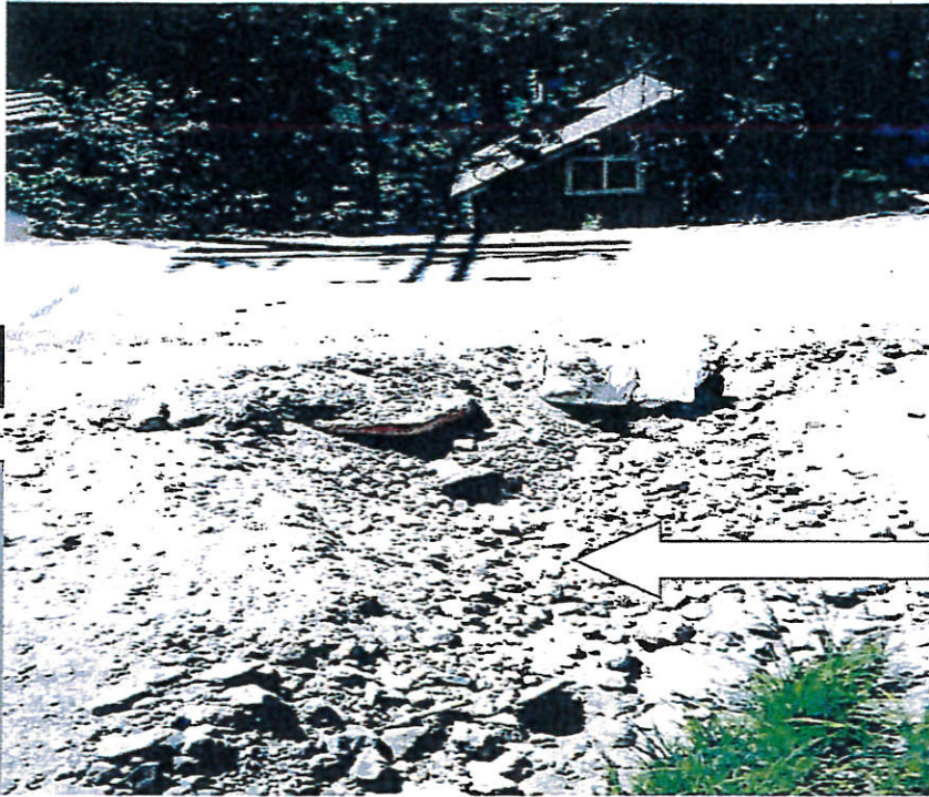
Photo 9. Culverts on the north shoulder of West Reed Avenue have been clogged by debris transported down the hillside. Photo taken May 29, 2006.
