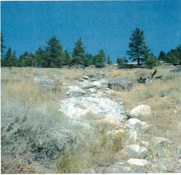
Channel characteristics downslope of I80 across bedrock material - looking upslope @ terminus of lower TDPUD access road.
