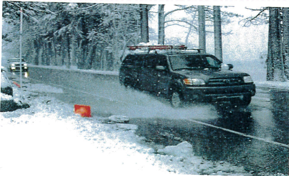
Photo 15. Between the residences of 15214 and 15234 Donner Pass Road runoff was observed sheeting across the road during several of the 2005/2006 rain storms (E. Kashtan, pers. comm. 2006). Vehicles kick up both water and erosion debris that can impact garages.
