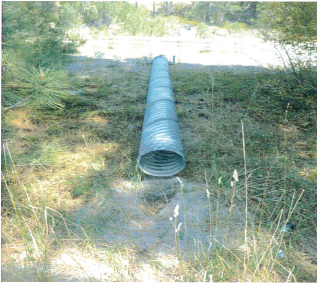
Terminus of culvert on west side of slope from east bound I80, does not drain into channel noted in photos below – flow is likely dispersed across landscape. Minimal erosion issues observed.
