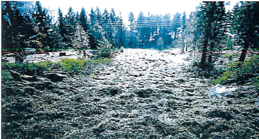
Photo 24. Erosion control measures were implemented on the site in September 2004 after the completion of construction. Photo taken October 2004.
