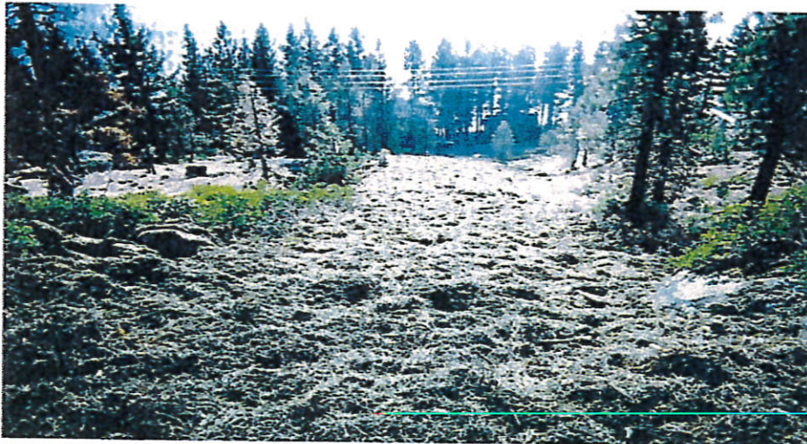
Photo 24. Erosion control measures were implemented on the site in September 2004 after the completion of construction. Photo taken October 2004.
