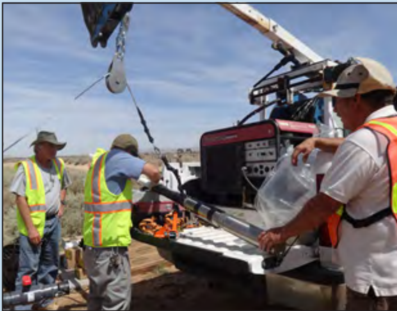
Figure 8. U.S. Geological Survey field crew preparing to set a temporary pump for borehole-geophysical data collection in a well, Hinkley, California, June 2015 (Roger Killian, Hinkley Technical Working Group, in foreground).
