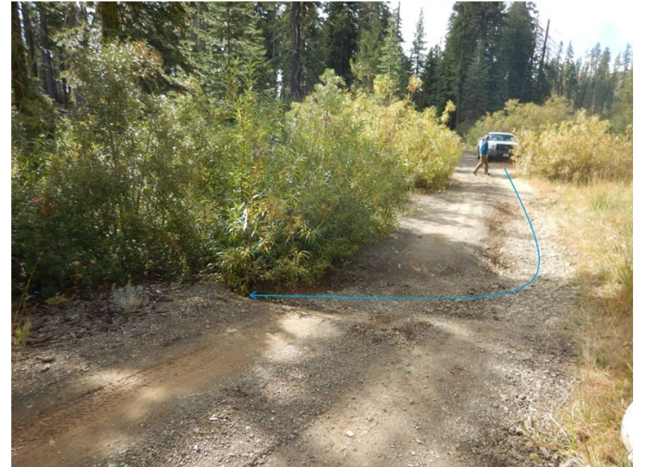
Photo 15. Road surface run off resulting in erosion and sediment delivery to an ephemeral watercourse.
