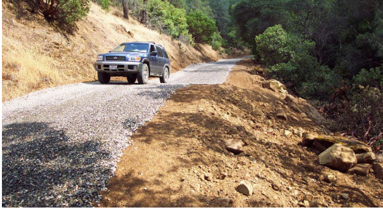
Photo 1. A rolling dip constructed on a rock surfaced rural road.
