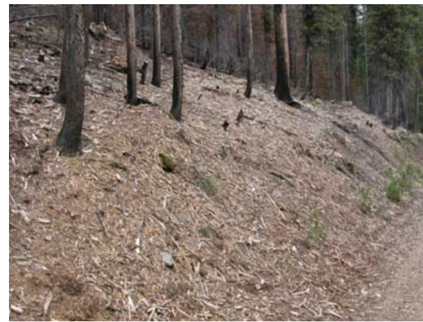
Photo 4. Mulch spread over a burned slope for erosion protection.
