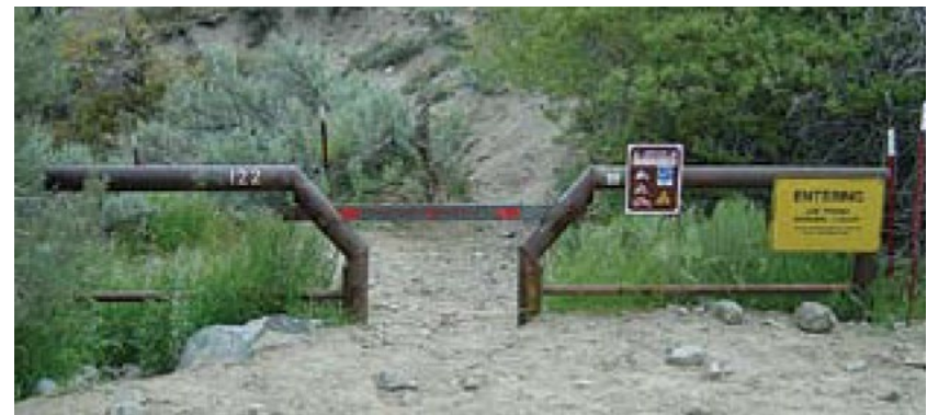
Photo 6. A vehicle access barrier.
