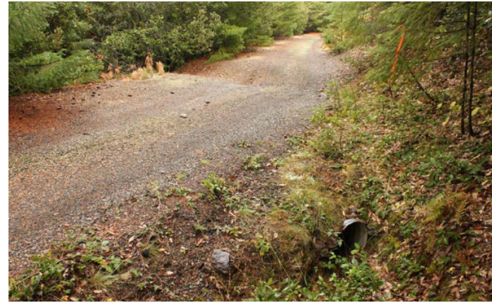
Photo 2. A waterbar on an unsurfaced road.
