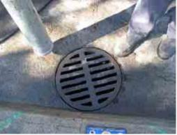
7b. Grate cleaned and replaced
