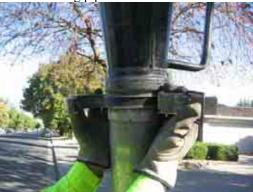
3d. Securing pipe to reducer cone
