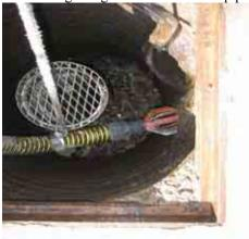
14c. Remove nozzle out of cross pipe
