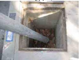
12a. Install pipes into catch basins
