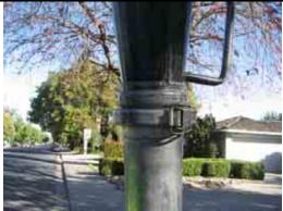
3e. Pipe secured to cone with clamp.
