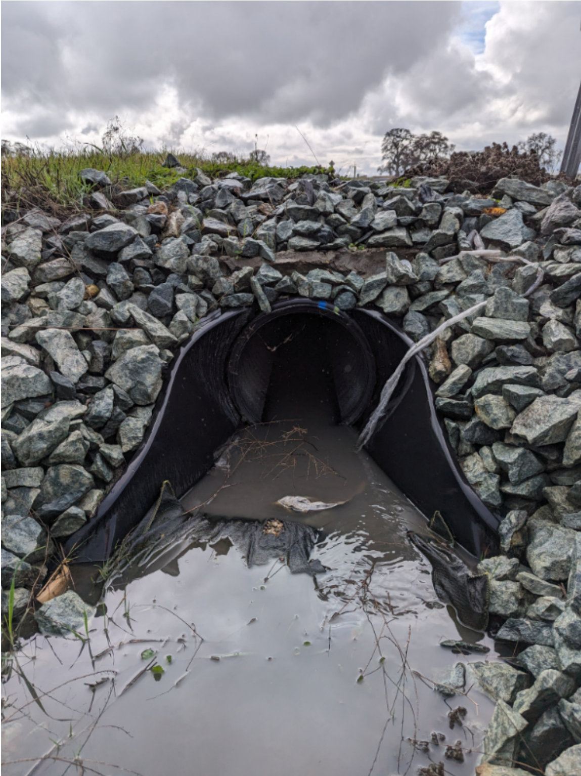
Figure 2: Existing Culvert, from North Side
