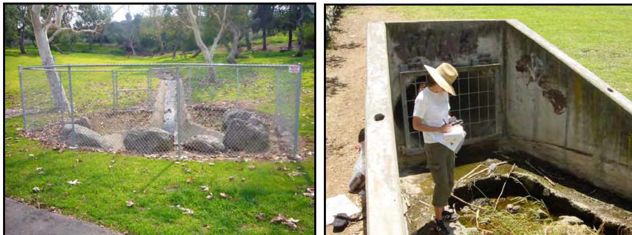
Figure 10-6. Storm Drain Discharges to Puddingstone Reservoir
