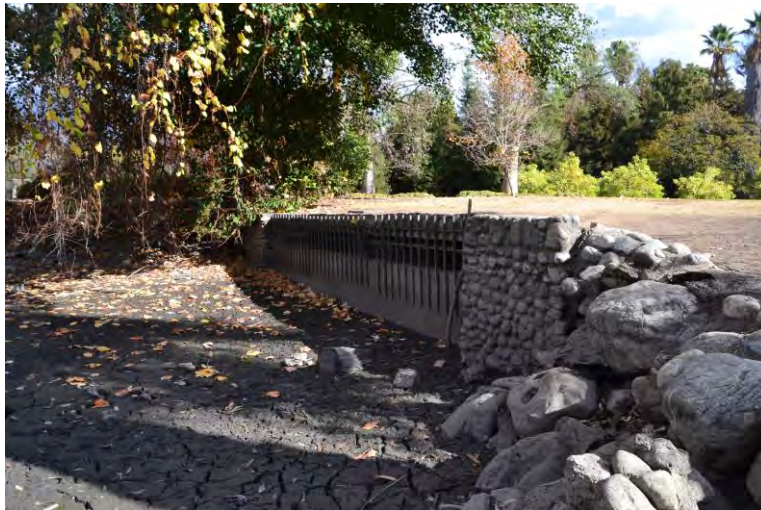
Figure 4. Tule Pond Existing Conditions and Outlet Structure
