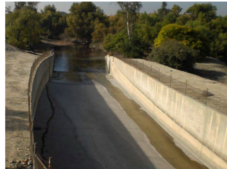
Sawpit Wash (Corps Built Channel)
