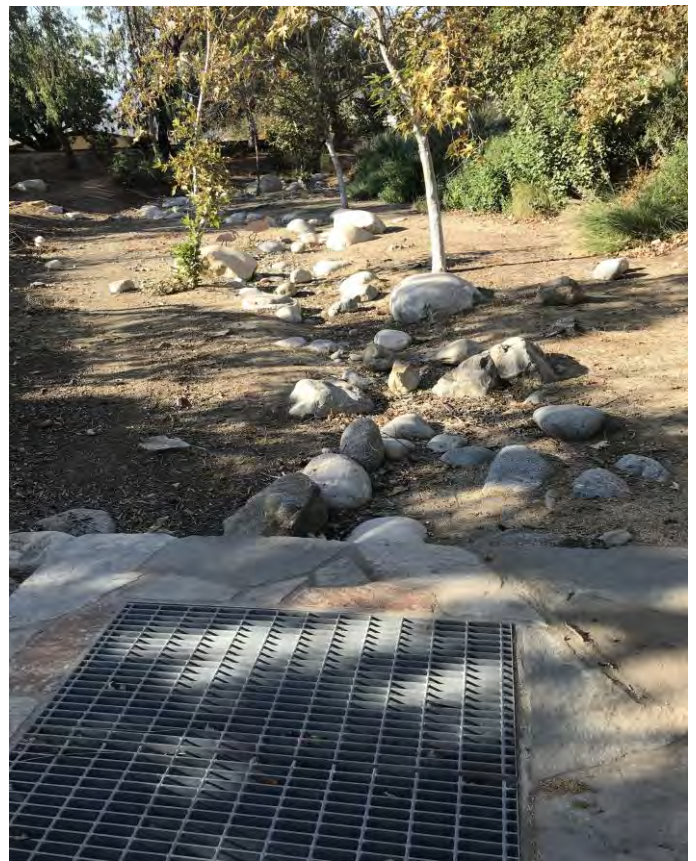
Figure 4. Grate Inlet at Downstream End of Natural Drainage Swale
