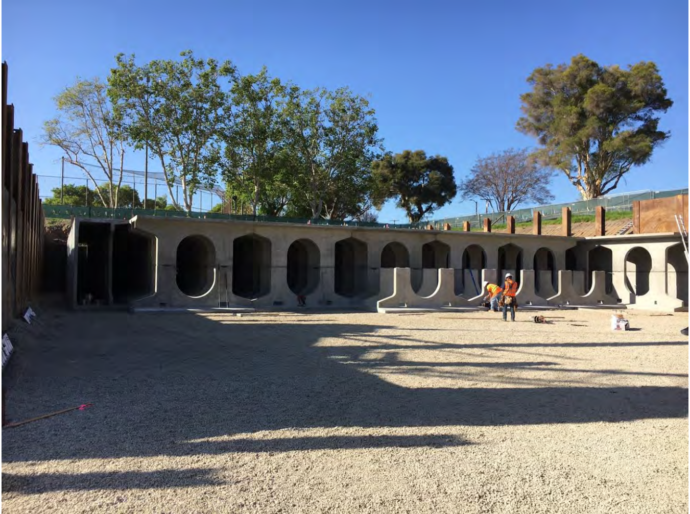
Figure 10. StormTrap Installation ad Bolivar Park BMP
