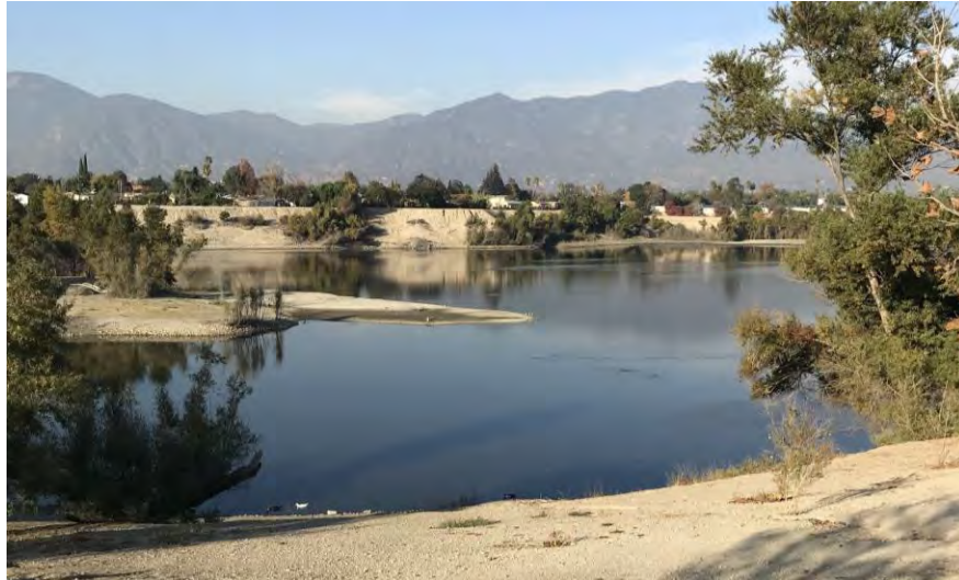
Figure 3. North Spreading Basin Looking Towards Sawpit Wash Inlet
