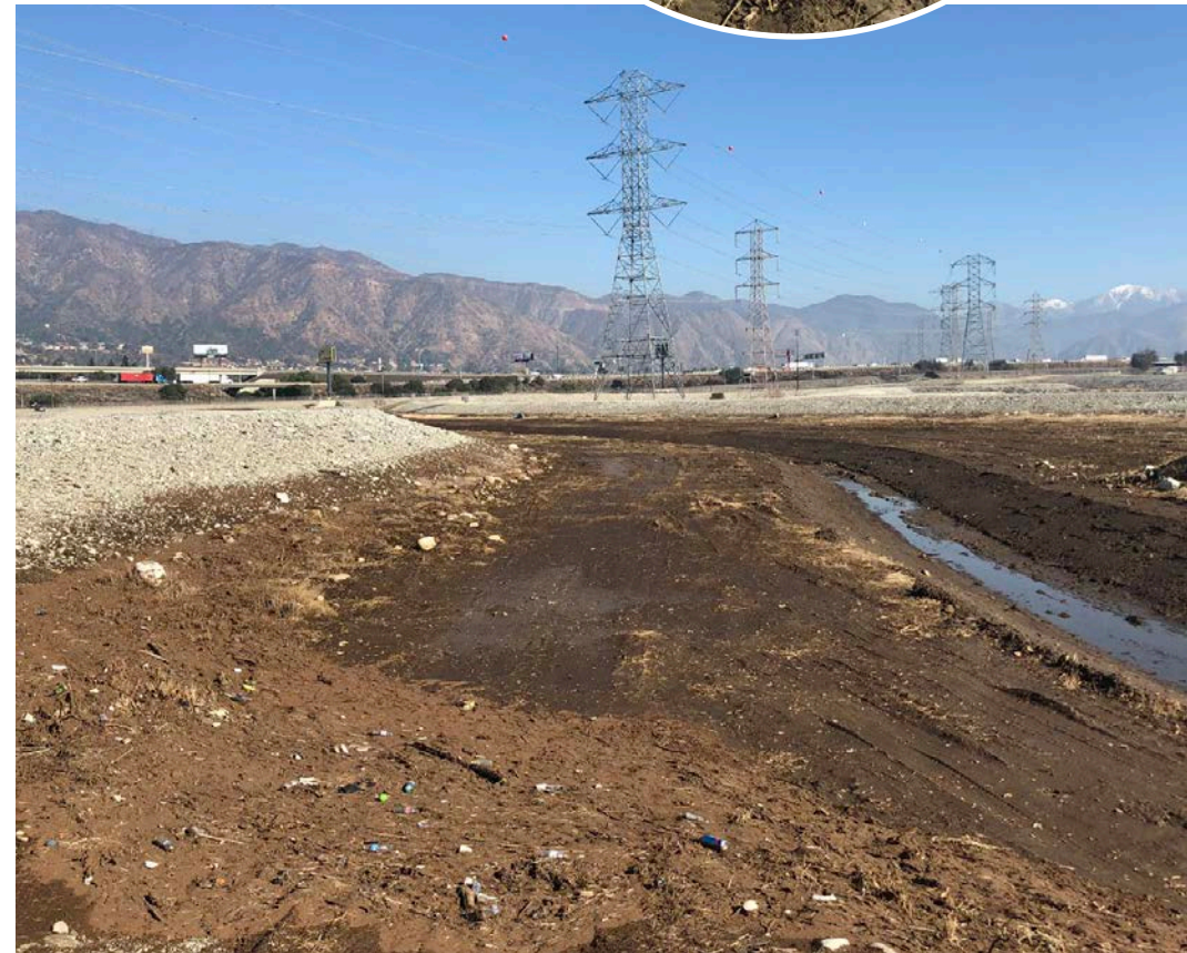
Downstream End of Basin 3E
