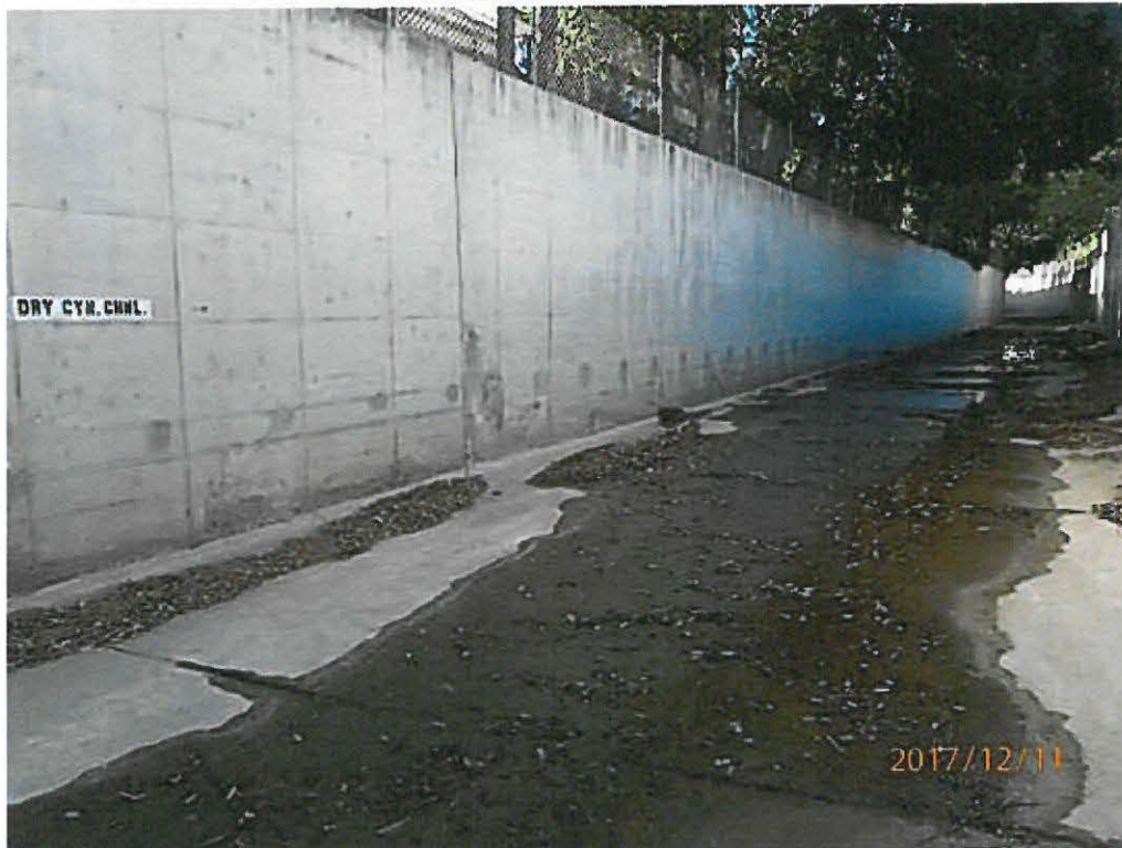
DCC_VEN Ground-Level View
