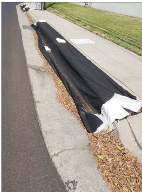
Figure 14. Catch basins along the study routes were covered to prevent trash from being swept into them.
