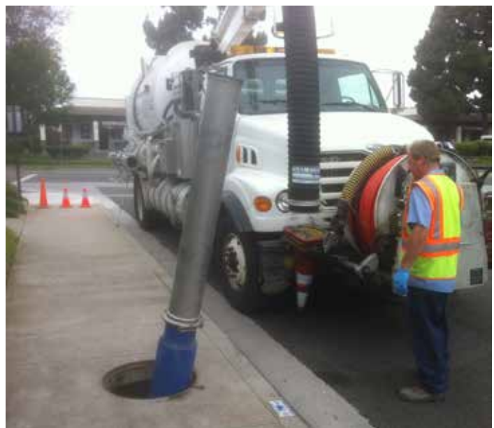
Catch Basin Cleaning Using a Vacuum Truck
