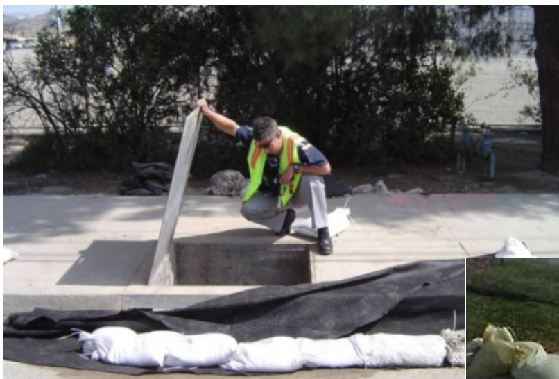
Inspection of catch basin BMPs
