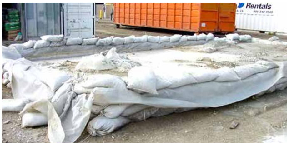
Concrete washout at construction site
