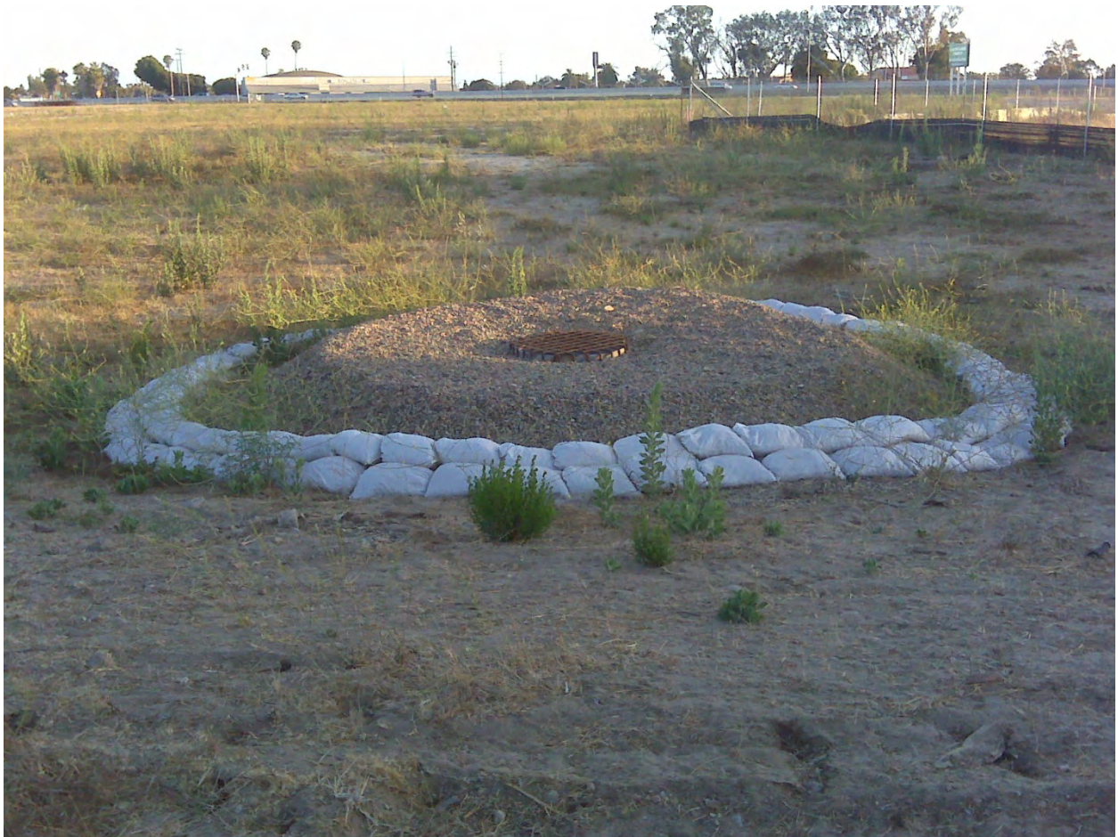
Storm drain protection during construction
