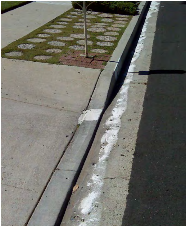
Evidence of an illicit discharge
