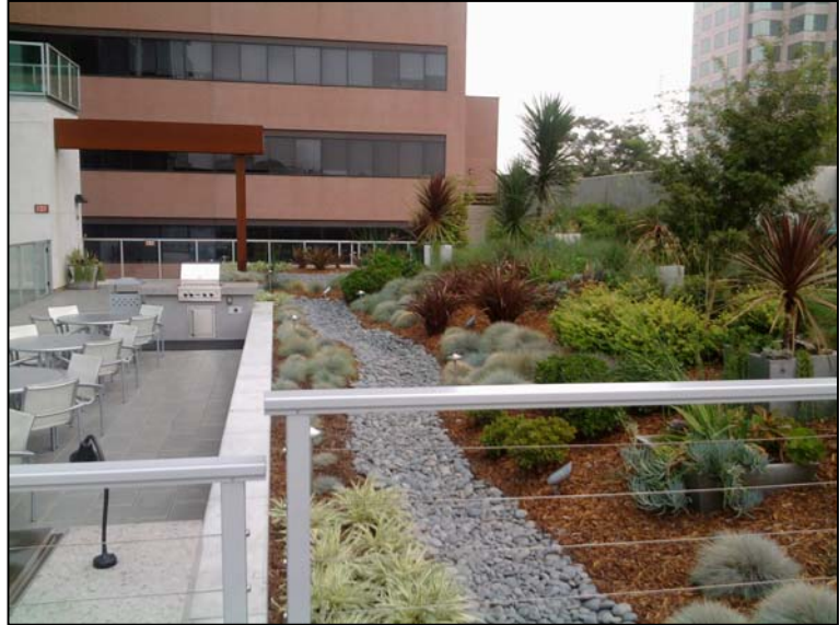
Bioretention (Planter Boxes)
