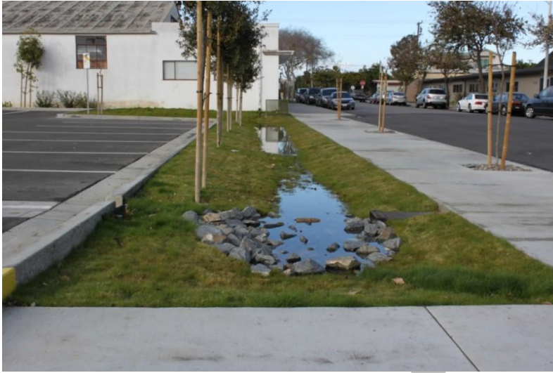
Figure 8: Vegetated swale (Signal Hill, CA).
