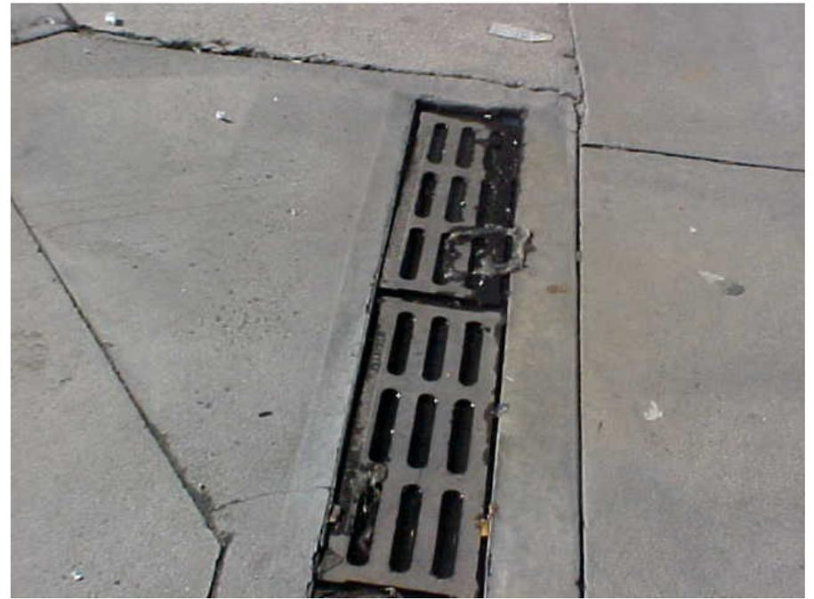
*Trench drain clogged with sediment*
