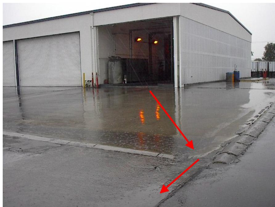
*The open corner of the partly contained area would enable wash water to flow outside the contained area*
