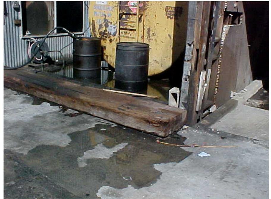
*Secondary containment structure overflowing*
