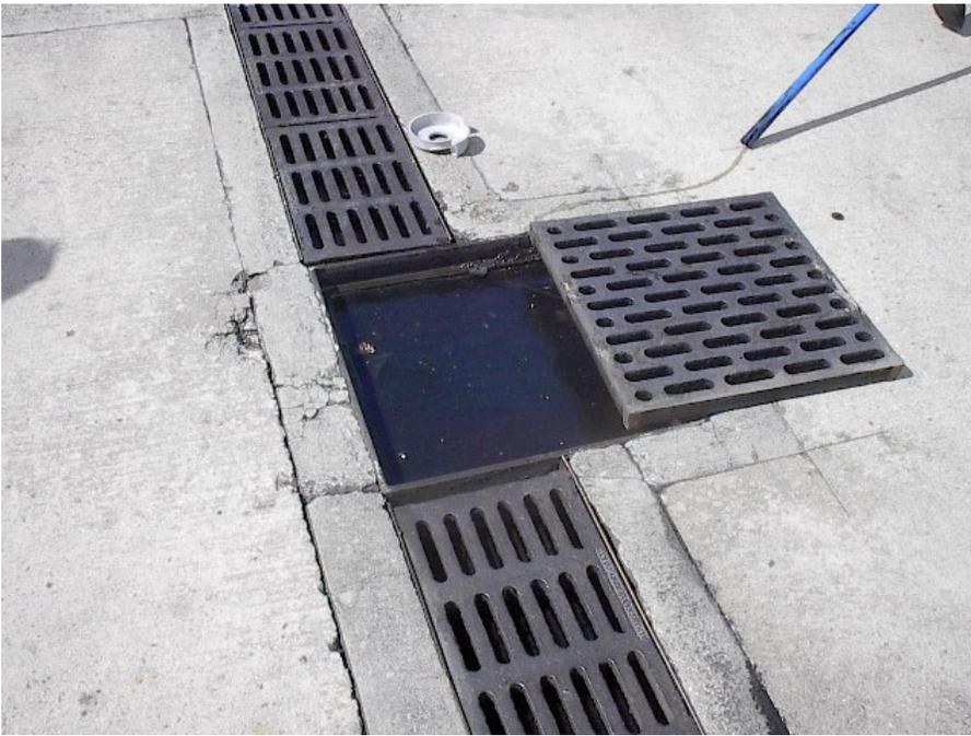
*Sump connection to the sanitary sewer was clogged*
