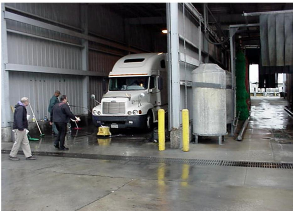
*Covered wash rack contained by slot drains*
