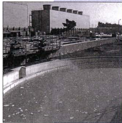
Sewage treatment plant in Orange County
