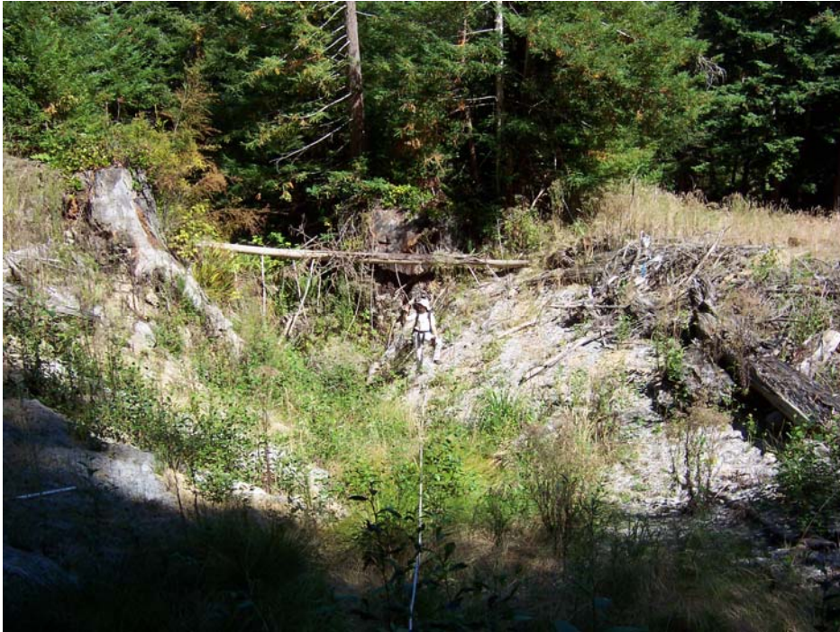
Appendix G. Headwaters Forest road r07, crossing 3 photo, September 4, 2004.
