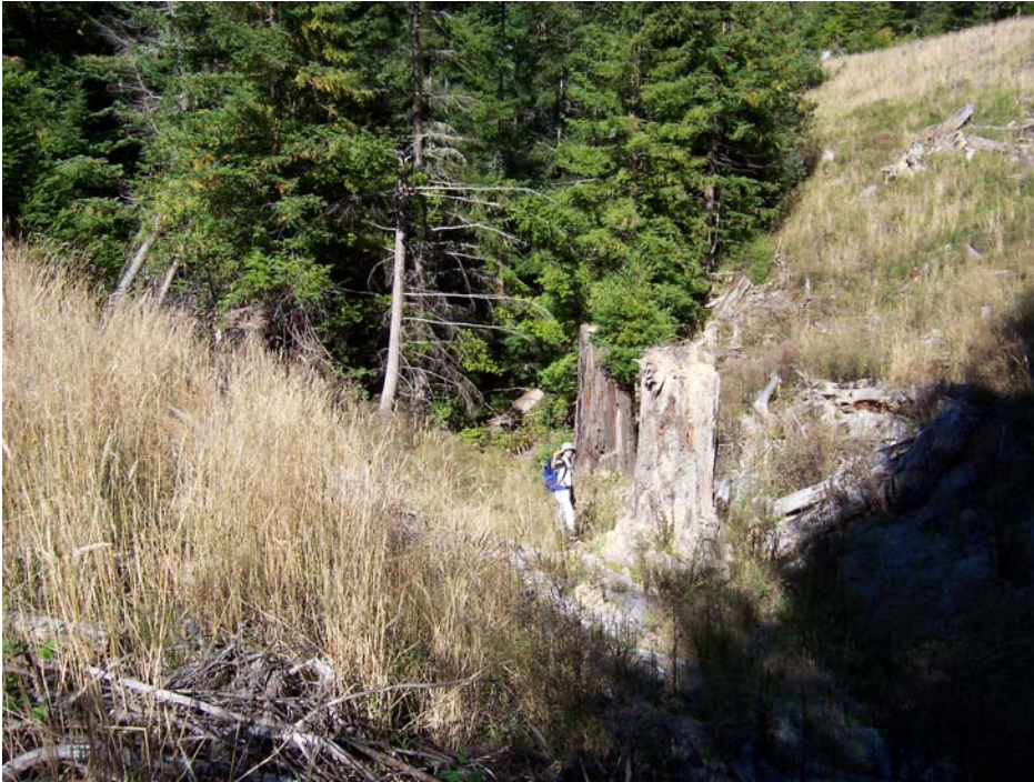
Appendix K. Headwaters Forest road r07, crossing 1 photo, September 4, 2004.
