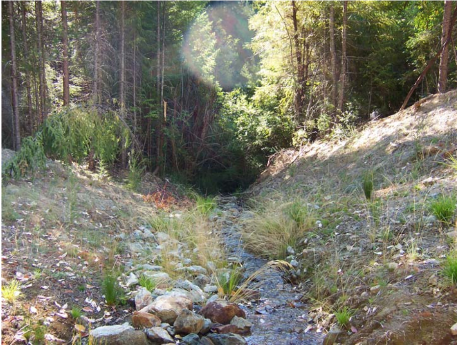
Appendix EE. Klamath Forest road 13N10, crossing 2 photo, August 18, 2004.
