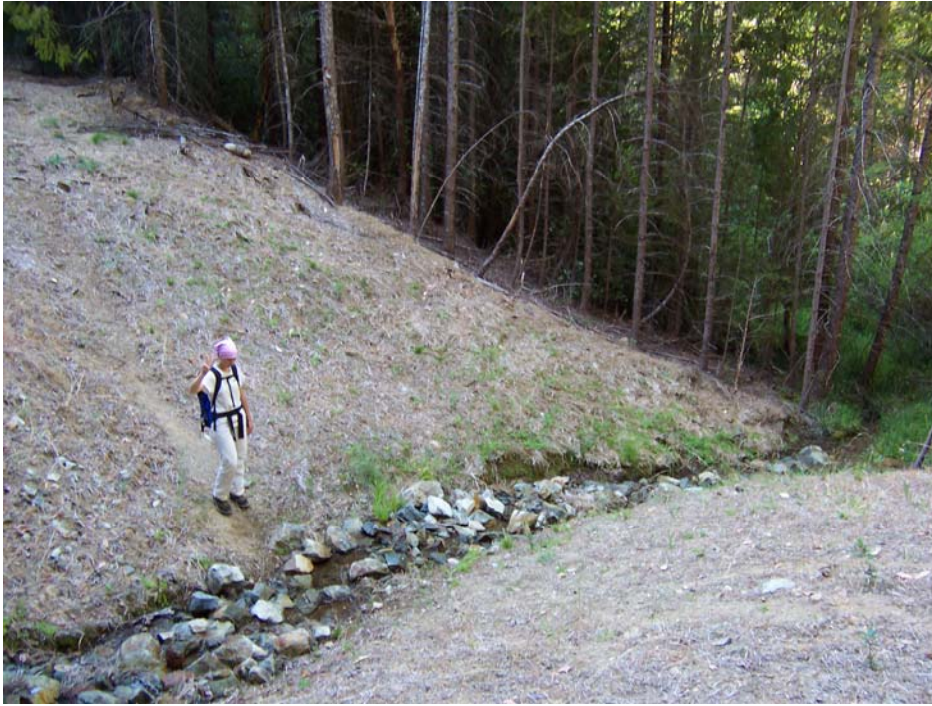
Appendix GG. Klamath Forest road 13N10, crossing 1 photo, August 18, 2004.
