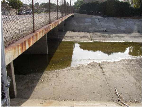
Figure D-5. Dry Weather Flow at the Los Cerritos Monitoring Station
