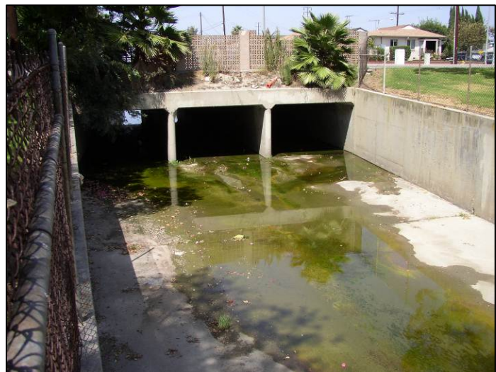
Figure D-3. Typical Dry Season Growth, Del Amo Channel.
