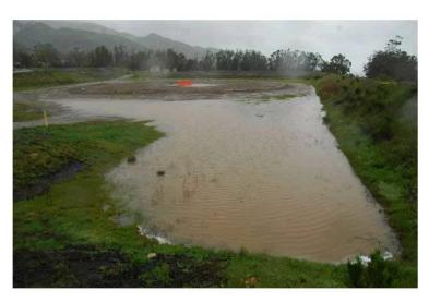
**Figure 5.** Former tank site with containment area at the Gaviota Terminal in Santa Barbara County during site remediation.
