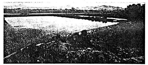
PHOTO 3 - Santa Rosa Sewer Farm showing south settling ponds with aquatic vegetation harboring mosquito breeding.
