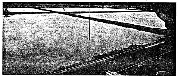
PHOTO 16 - Sebastopol Sewage Disposal Plant. Sludge drying bods and oxidation ponds. Effluent from latter to Laguna at farthest corner in right distance.
