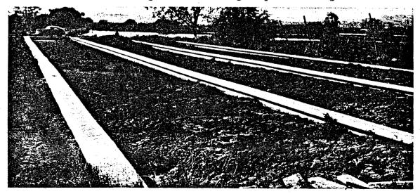
PHOTO 4 - Santa Rosa Sewer Farm showing concrete settling tanks with crust.
