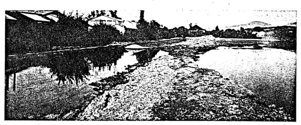
PHOTO 14 - Effluent pond Healdsburg Dehydrating Plant, processing potatoes and carrots. High organic content and very odoriferous. Pond on left has overflowed onto field at right.
