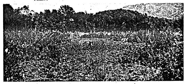
PHOTO 20 - Seepage Basin for effluent of Imhoff tank at Cloverdale Sewage Disposal Plant.
