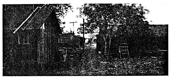
PHOTO 28 - Housing Unit reconstructed from chicken houses, one block west of City limits of Santa Rosa. Building at right, formerly a brooder house, has four rooms and is without windows.
