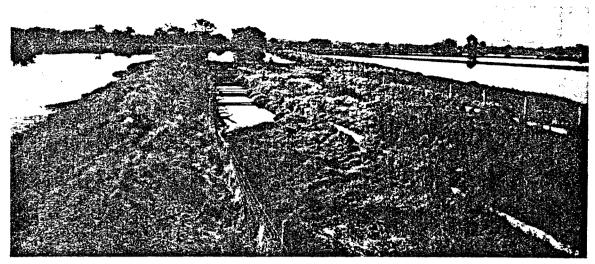
PHOTO 2 - Santa Rosa Sewer Farm showing wooden septic tanks. Two chlorinator houses appear as white square spots in distance.
