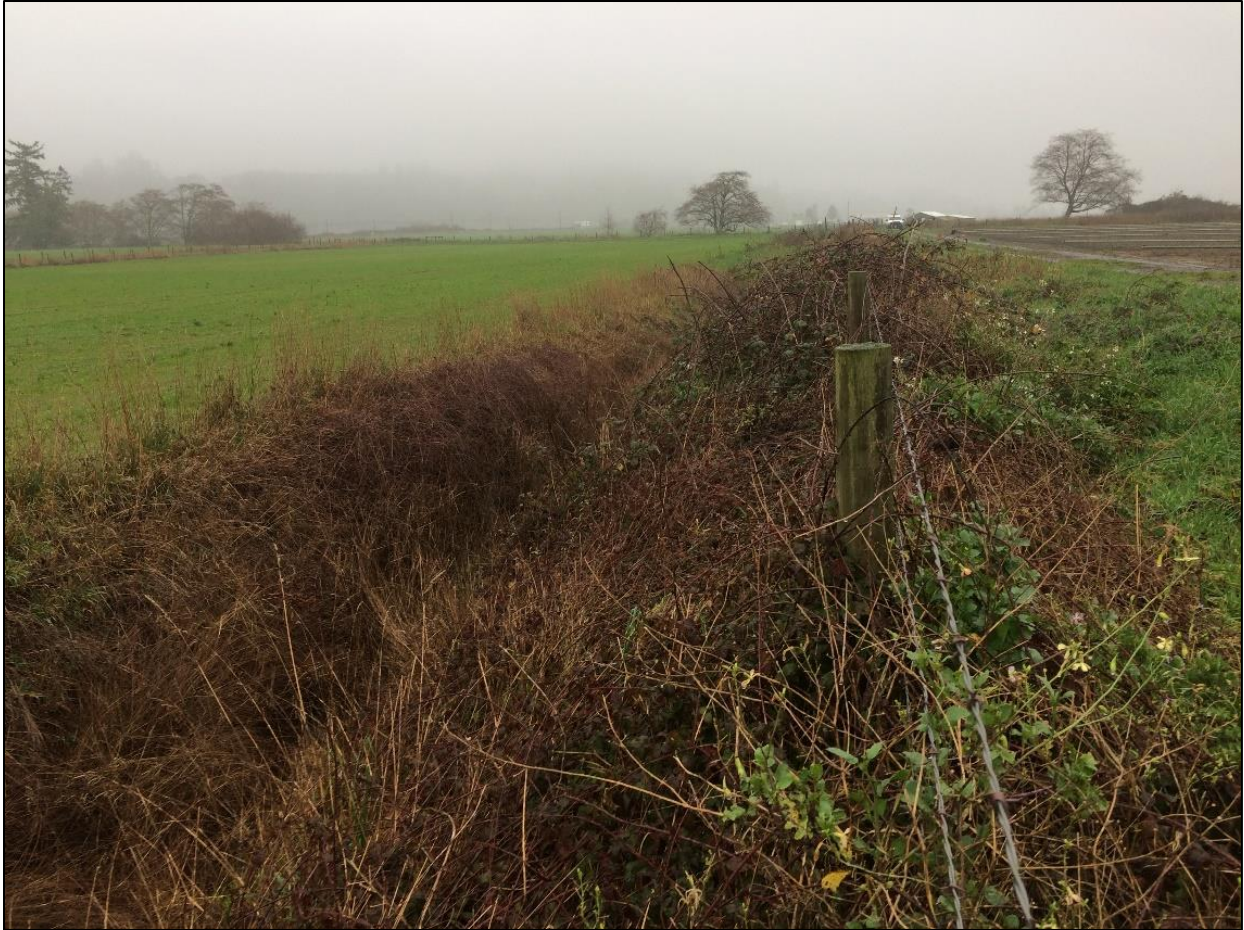
Figure 4.5. Grassed Waterway. Grass and other vegetation are maintained in this ditch to slow water, drop out sediment, and filter pollutants.
