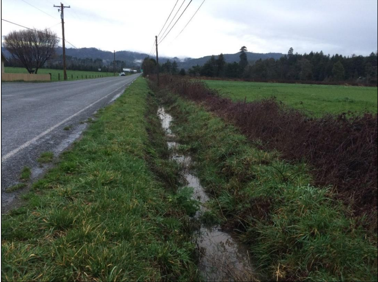
Figure 4.3. Grassed Waterway: A roadside ditch is maintained with vegetation growing on the bottom and side of the ditch. This slows water and allows sediment and any attached pesticides to settle.
