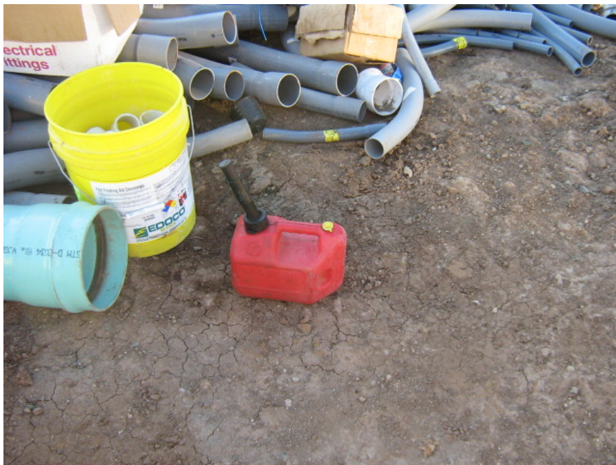
Photograph 4: A fuel can filled with gasoline was stored where it could be exposed to storm water contact
