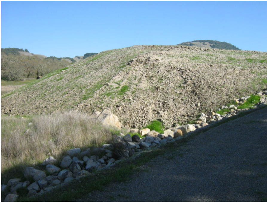
Photograph 13: Unstabilized soil stockpile area adjacent to the main access road
