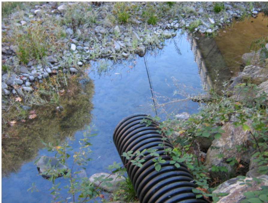
Photograph 18: Culvert pipe outfall to Matanzas Creek
