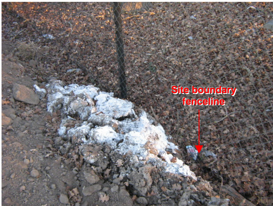
Photograph 6: Lime spillage and/or over-application was present where it could be discharged directly offsite
