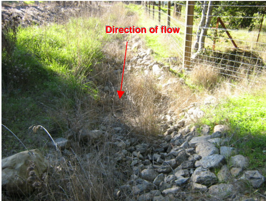
Photograph 17: View of roadside ditch leading to Matanzas Creek
