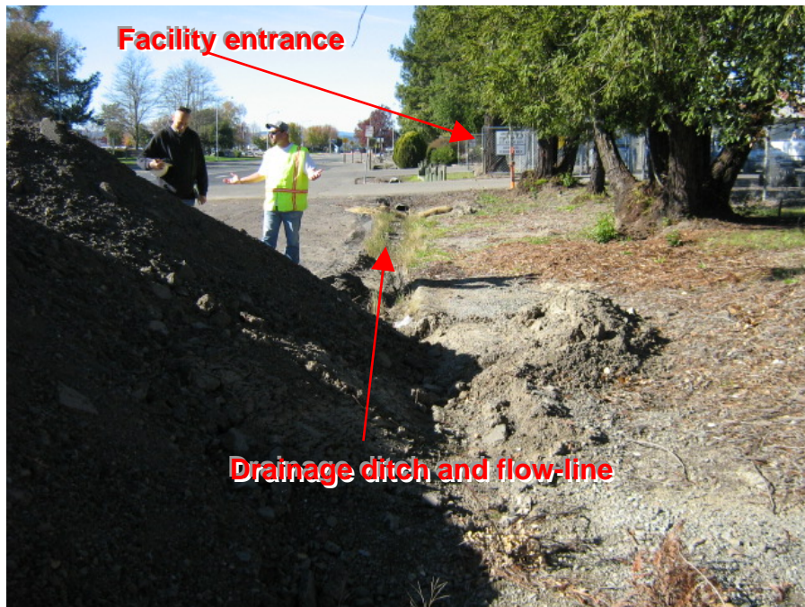
Photograph 24: View showing stockpiles and flow direction in the roadway drainage ditch
