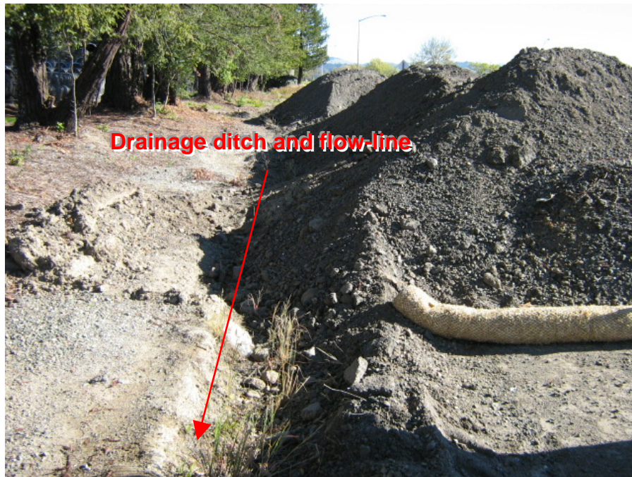
Photograph 23: Recycled asphalt stockpiles located in the roadway drainage ditch, a component of the MS4 drainage infrastructure
