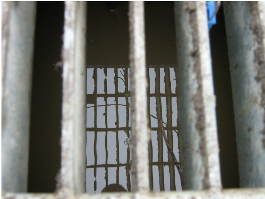
Photograph 24: Turbid water present in the storm drain inlet shown in the previous photograph
