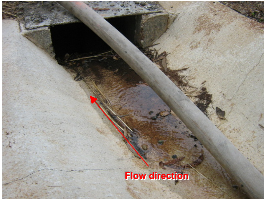
Photograph 17: Sediment and debris conveyed from the ditch and associated sediment controls into the down-gradient inlet
