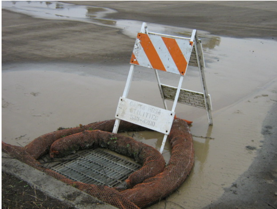
Photograph 23: Receiving inlet located down-gradient of the dump site and adjacent stockpile
