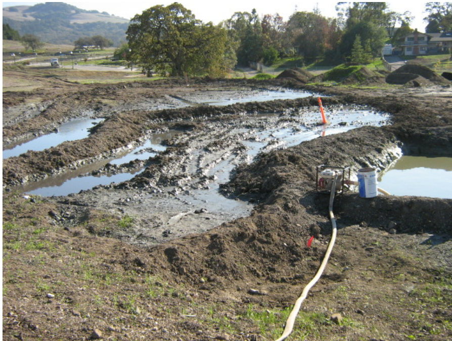
Photograph 2: Large expanse of unstabilized soil including the area where well drilling fluids had been applied
