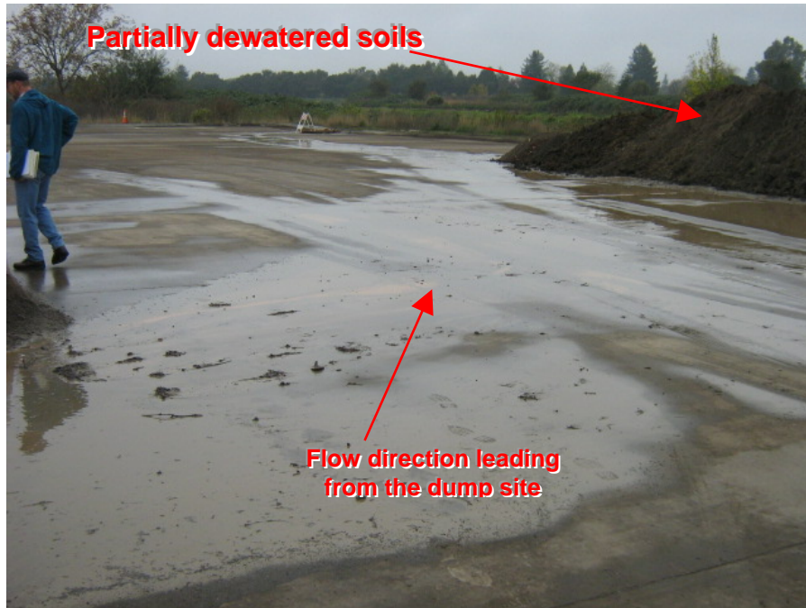
Photograph 21: Partially dewatered soils placed in the flow-line of the dump site
