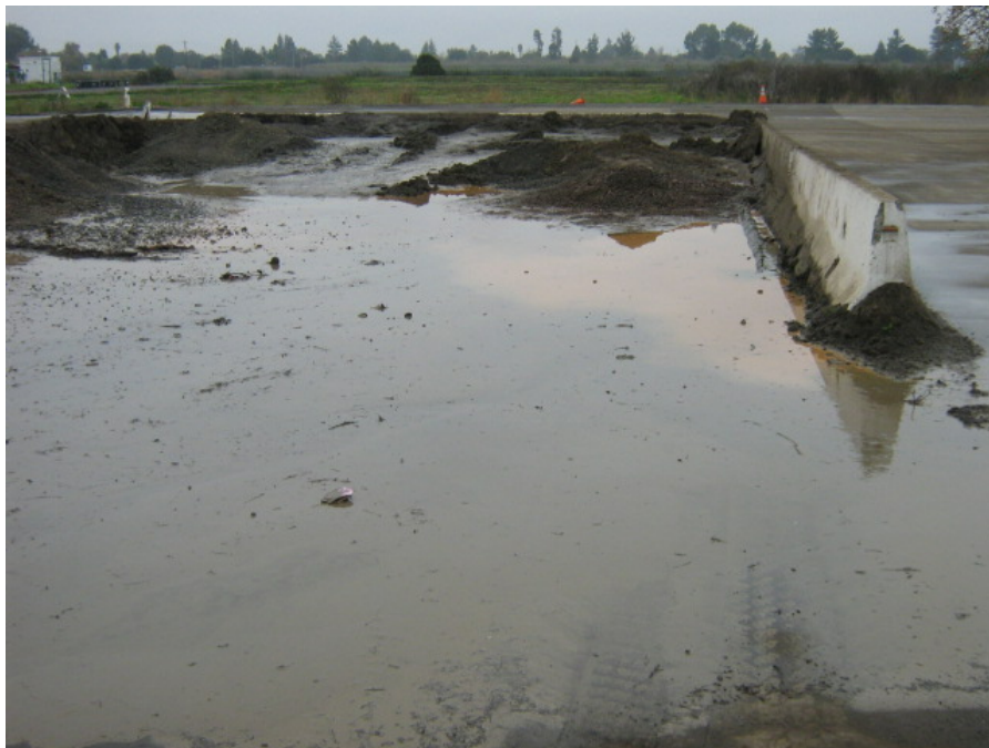
Photograph 20: Stockpile of saturated soils resulting from hydro excavation, which may be contaminated with sanitary waste
