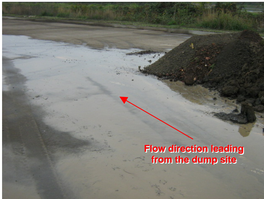
Photograph 22: Close-up view of turbid water flowing from the dump site and partially dewatered stockpile
