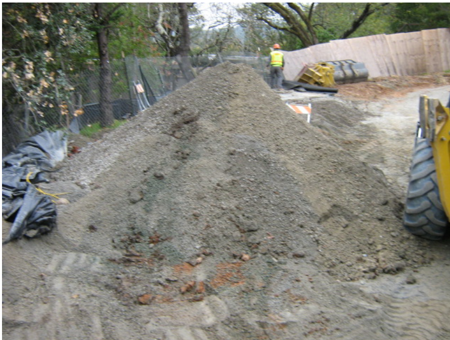
Photograph 10: Soil stockpile and area of unconsolidated material located on the down-gradient perimeter of the project site
