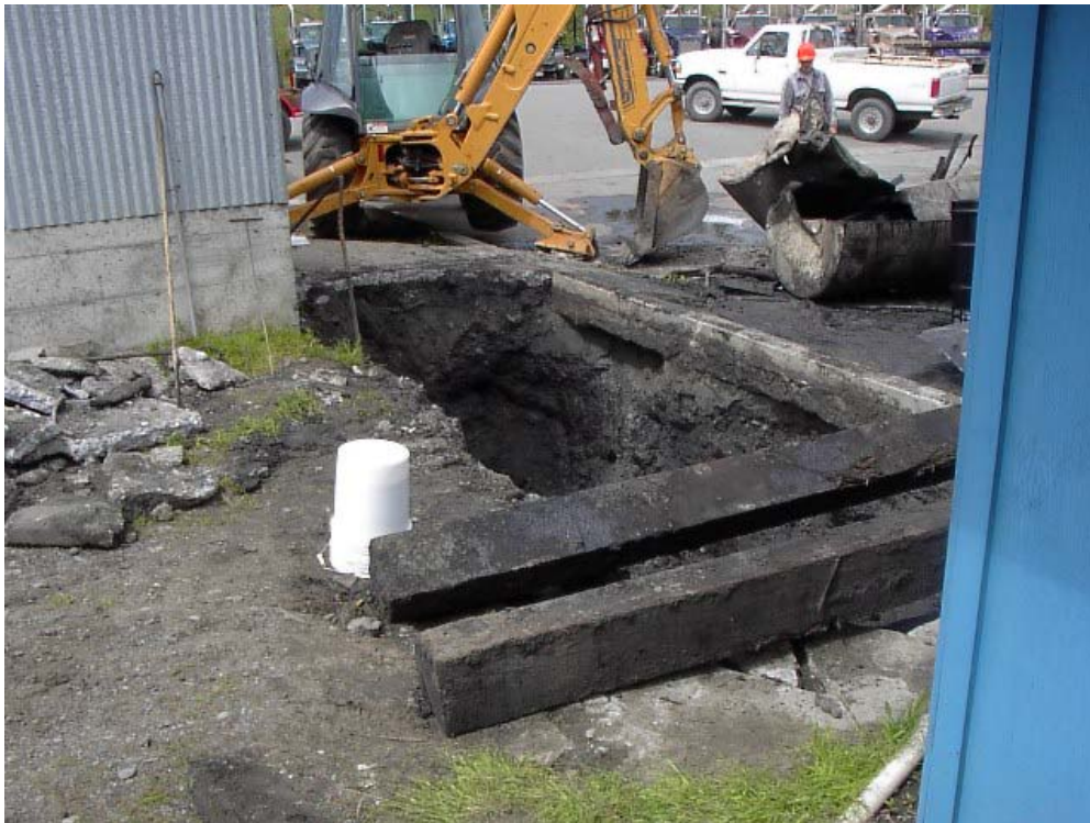
Waste Oil UST excavation.
