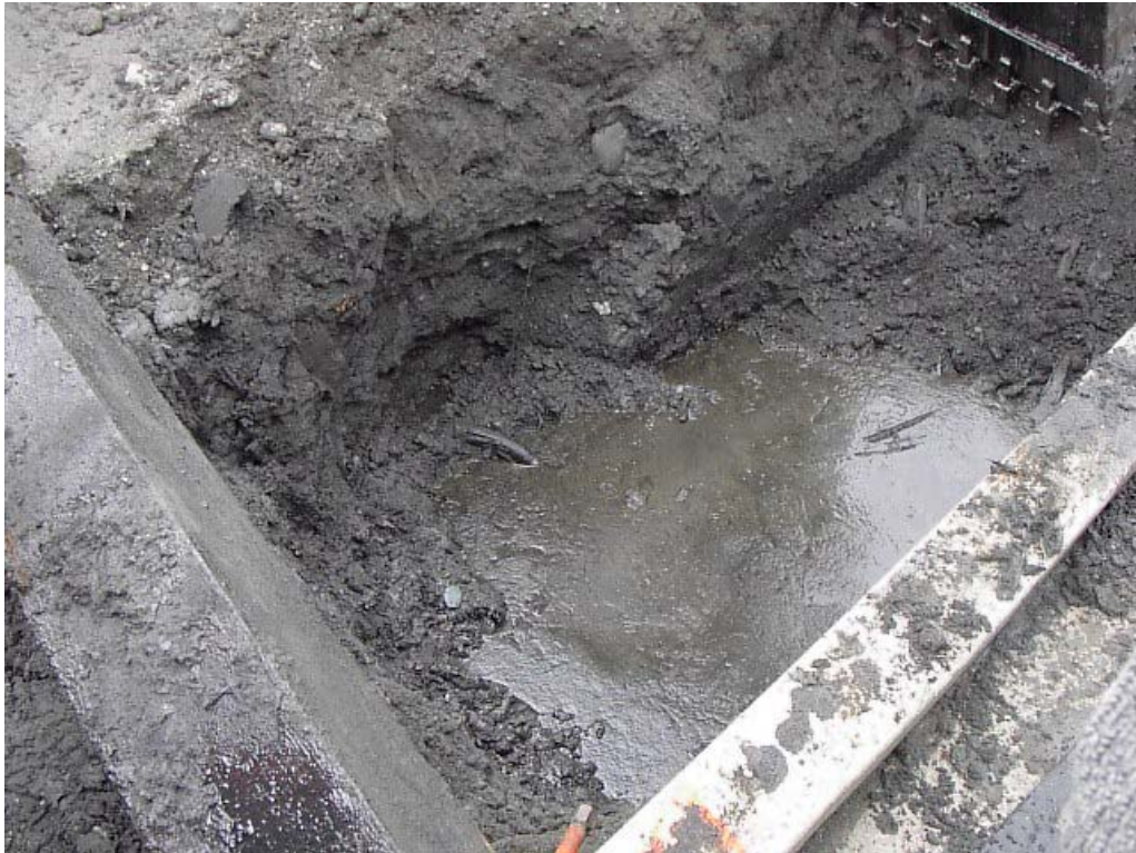
Groundwater in UST excavation encountered at approximately 5 feet below ground level.
