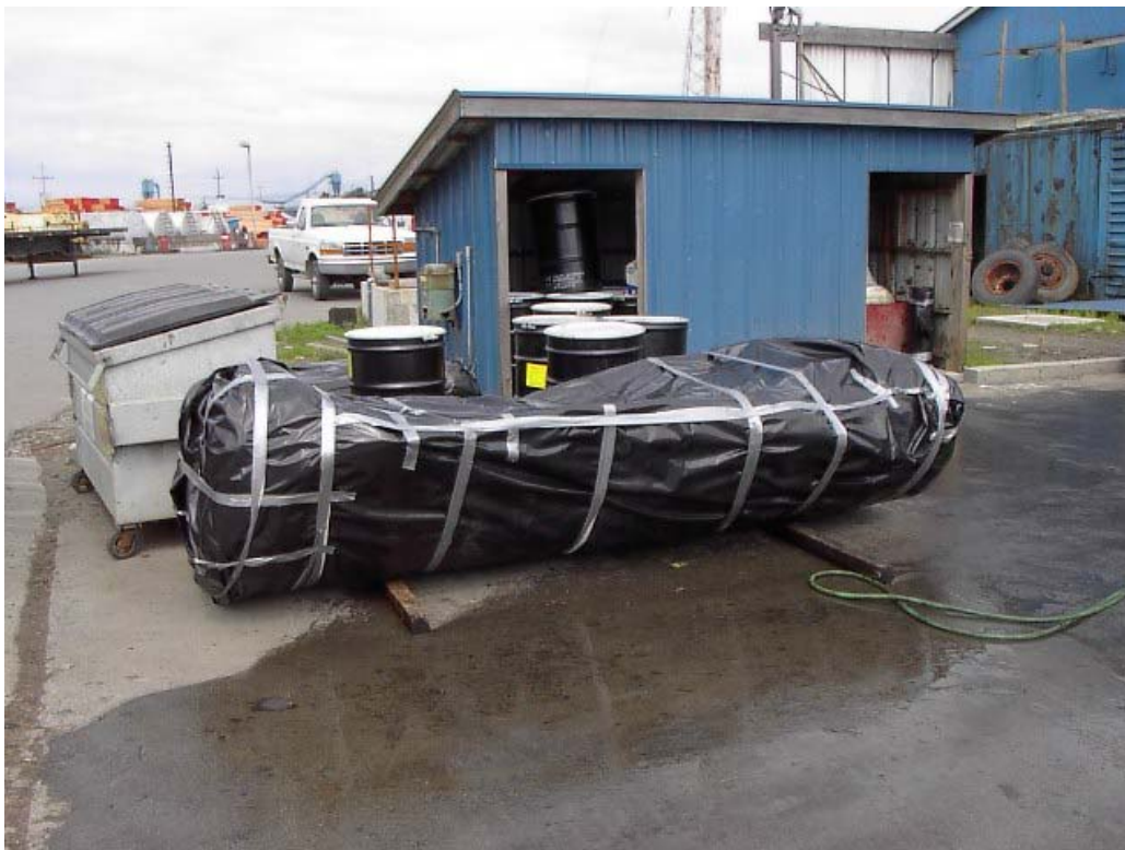
Picture looking east showing the UST prepared for transportation.
