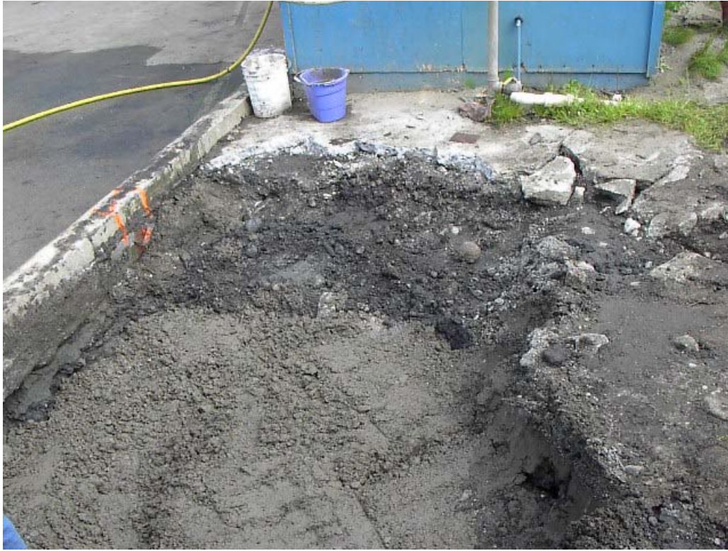
Picture looking southeast showing excavation with clean backfill material.
