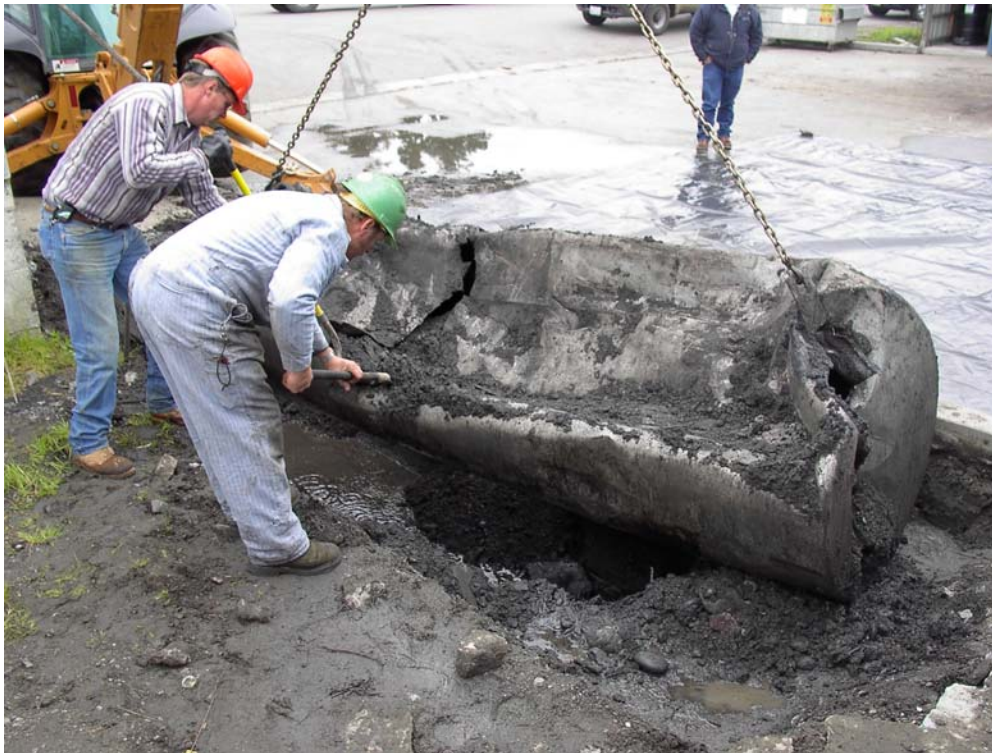
Removal of the Waste Oil Tank. UST was discovered crushed in-place.
