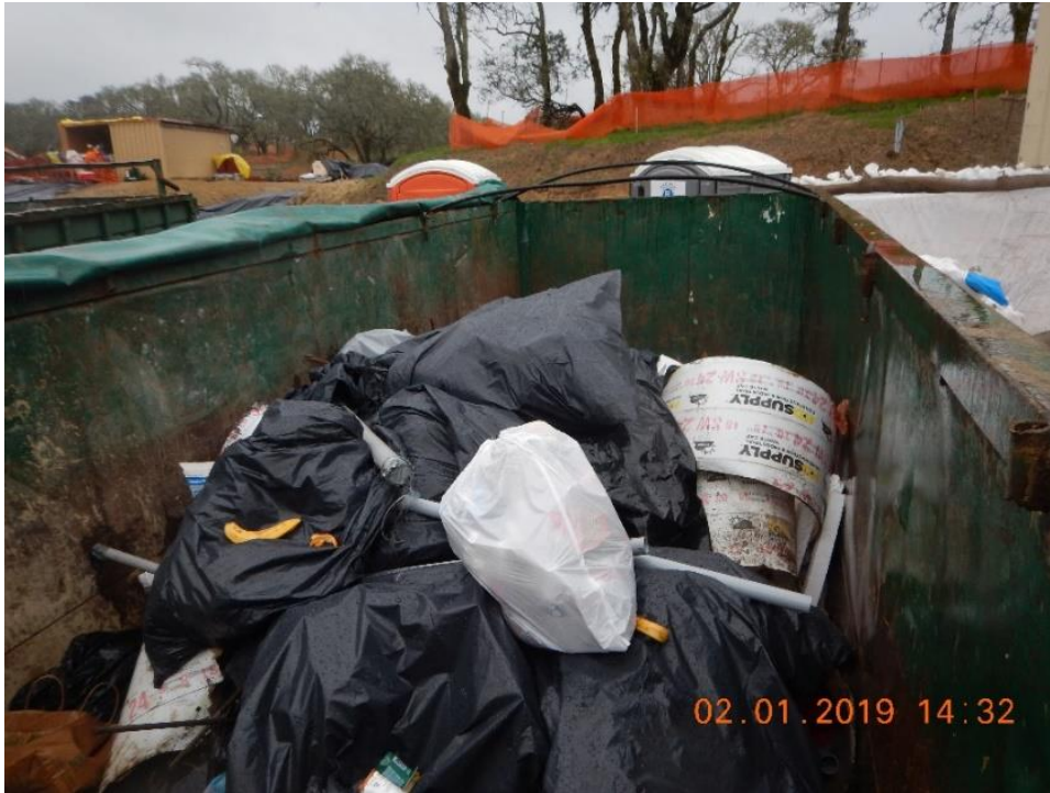
Figure 29. Partially filled waste bin, uncovered, during rainfall.
