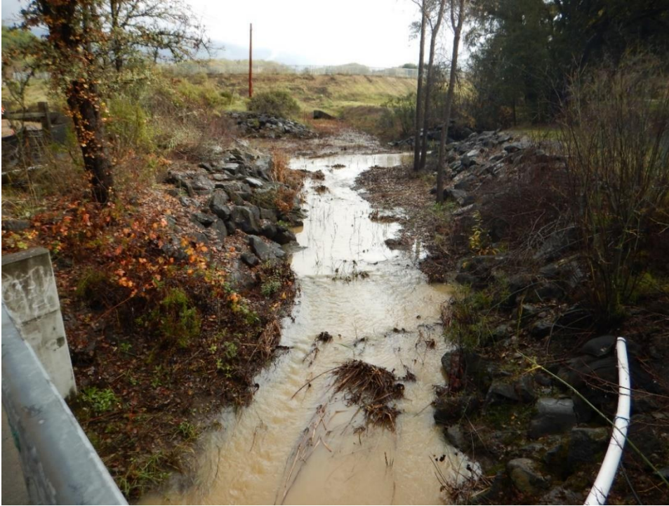
Figure 43. November 29, 2018. Foss Creek Bridge on Healdsburg Avenue downstream of Site. In route to the Site, staff noticed Foss Creek was highly turbid.
