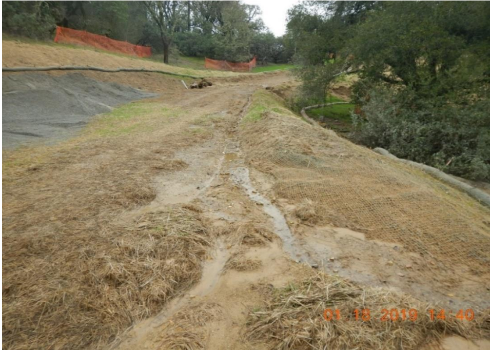
Figure 25. Lack of effective linear sediment controls at the toe or break in a slope.
