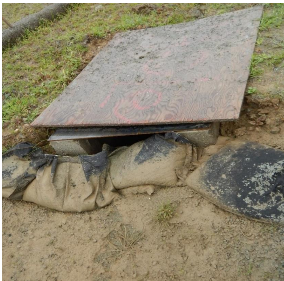
Figure 20. Farther downstream of Figure 19 above, the silt deposits show that sediment-laden water impounded sufficiently to overtop the center bag.
