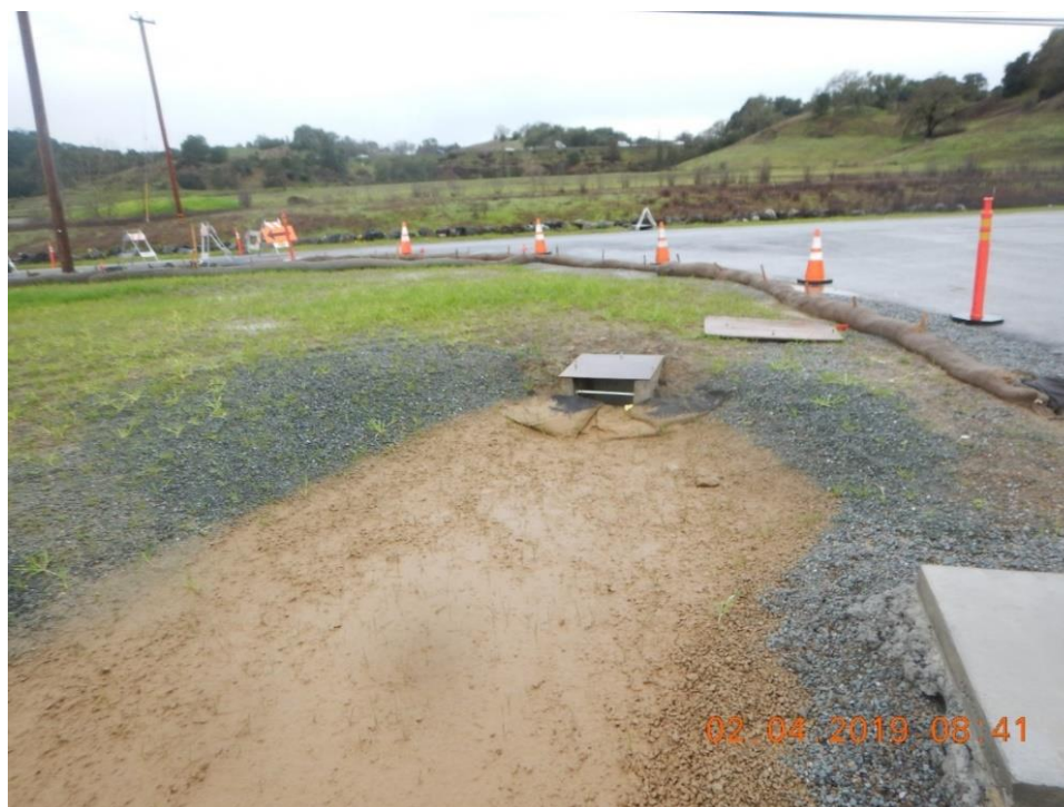
Figure 38. Downstream of Figure 37 above, sediment has overtopped the gravel bags and discharged sediment-laden runoff to the storm drain system that discharges to Foss Creek.
