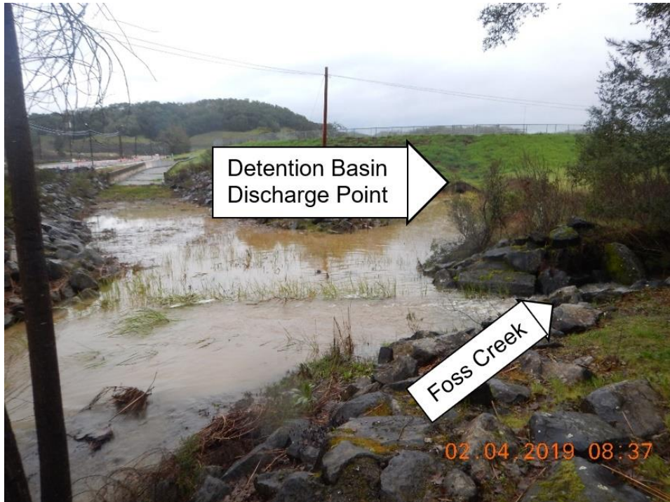
Figure 42. Discharge point from the City's detention basin which is receiving flow from the Site and delivering turbid water to Foss Creek.
