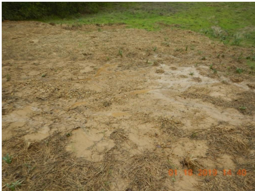
Figure 24. Lack of perimeter controls downhill from disturbed soil areas.
