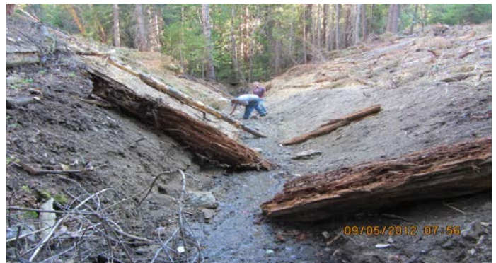
A larger crossing: Note the use of wood to control flow velocities. (Feiler 9/5/2012)
