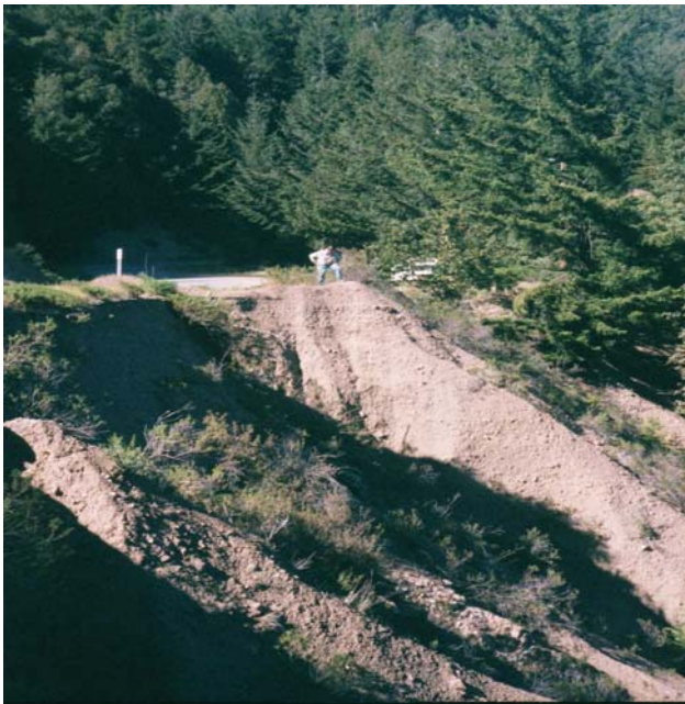
Figure 1. Road-related landslide.
