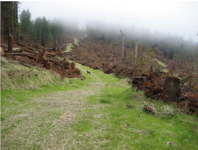
Figure 4. Recent shovel logging adjacent to newly constructed and reconstructed, mulched road surface. Note the extensive ground cover on the recent cut areas.
