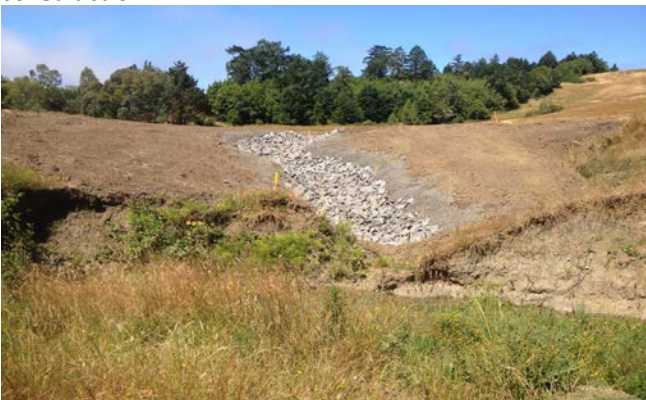
Photo 4: South gully looking upstream at final grade with rock placed.
