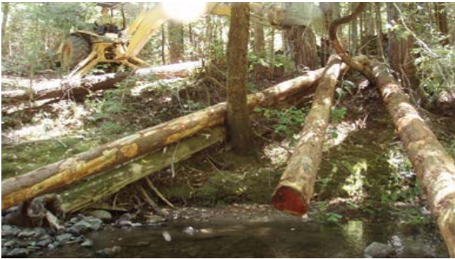
Figure 2: Ken Smith weaving large wood into a fish-bearing watercourse. Photo credit: David Wright, TNC.
