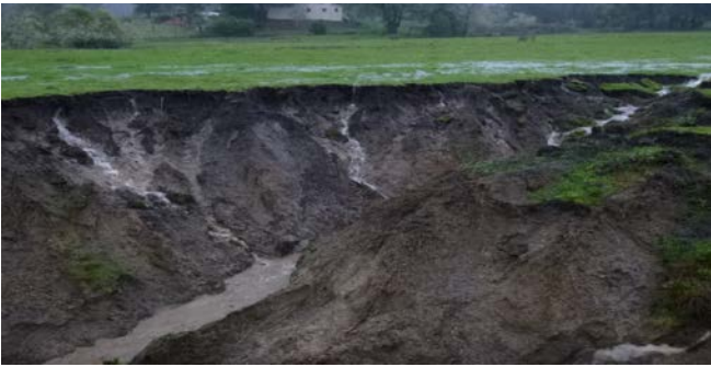
Photo 2: South gully looking upstream during a rainstorm in the winter of 2016-17.
