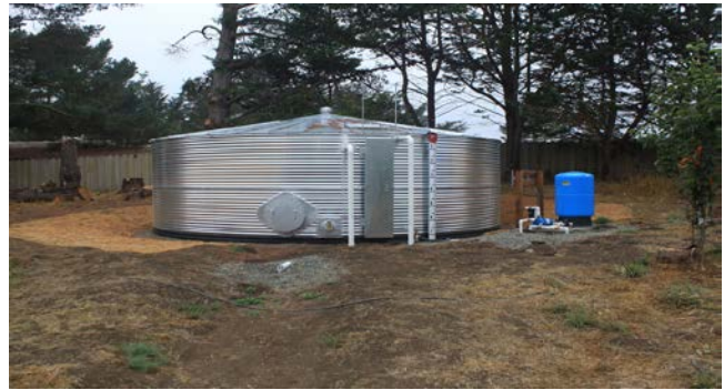
Photo 11: The completed 25,000-gallon tank installation.
