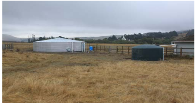
Photo 12: The completed 50,000-gallon tank with pump and pressure tank.
