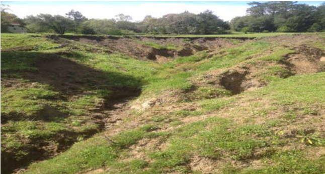
Photo 3: South Gully looking upstream, before project construction
