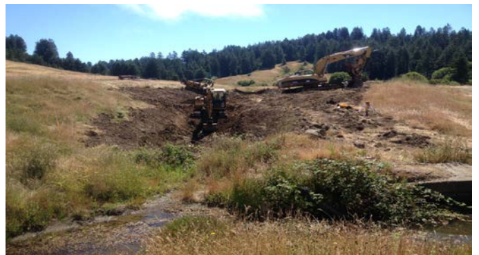
Photo 8: Start of excavation on the East gully looking upstream.
