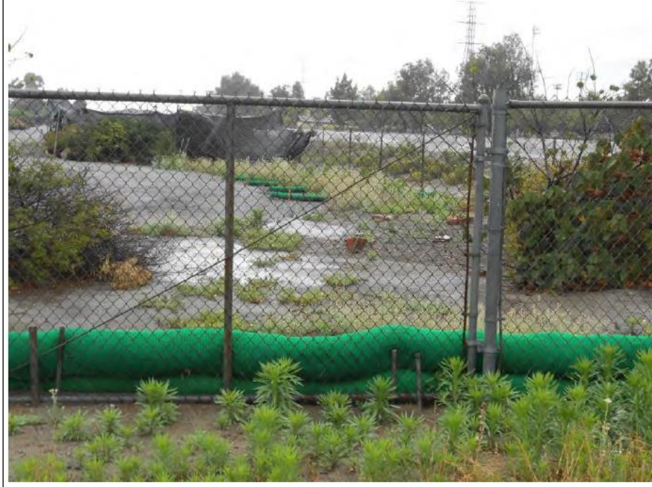
Figure 35 Filter Sox installed at San Gabriel River Nursery retains stormwater runoff from site
