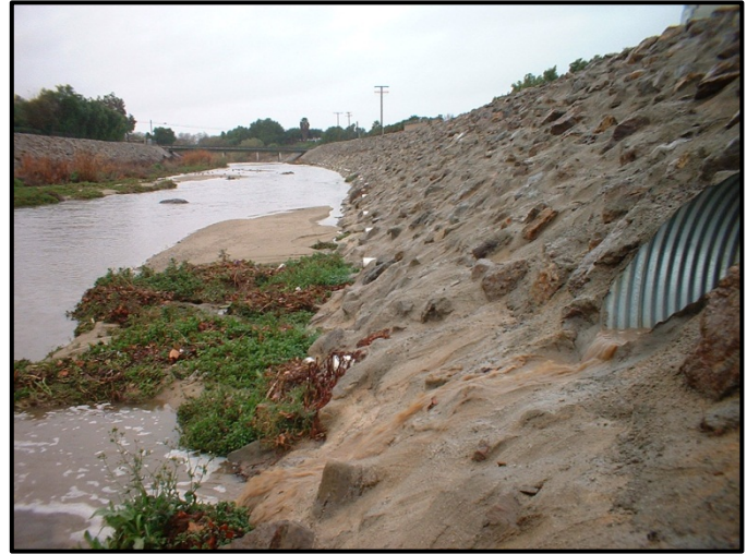
View of pipe discharging into Arroyo Simi
