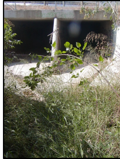
View of site (S) toward Hwy 126
