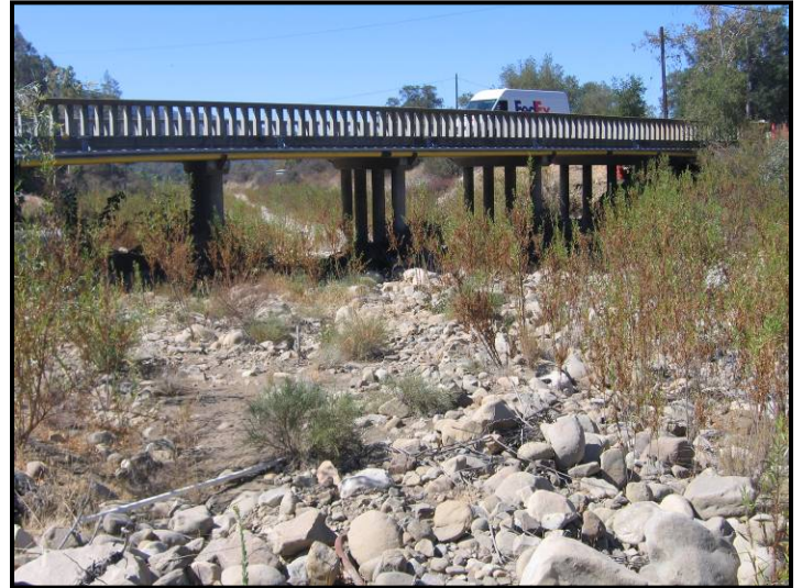
View downstream at the Grand Ave. bridge
