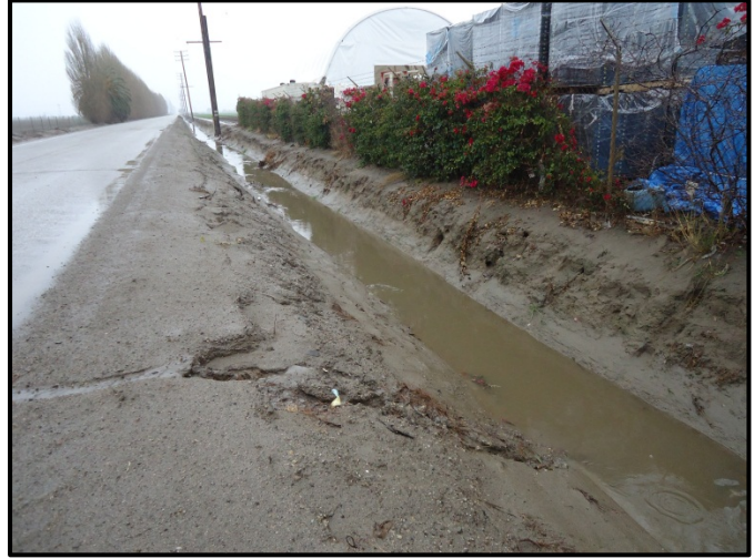
View at site looking upstream
