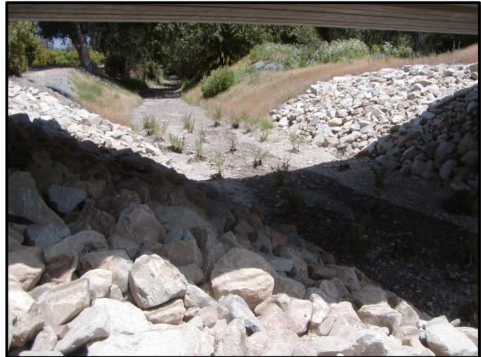
View upstream at the bridge
