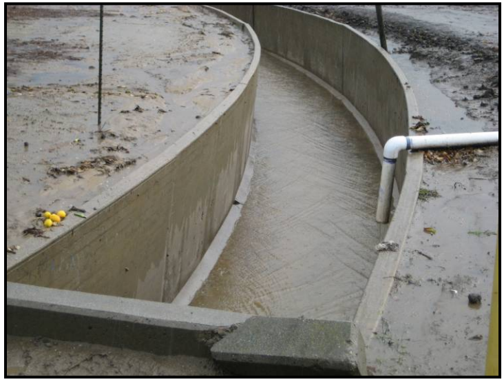
View upstream (NE) from sampling location
