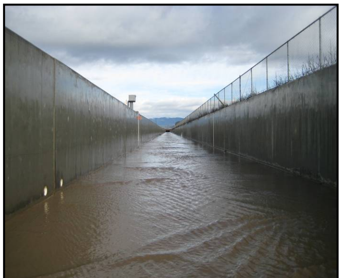
View upstream (NW) facing gage #781
