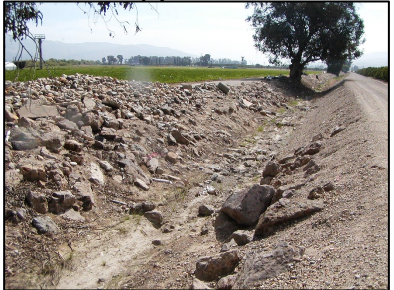
View of site looking upstream
