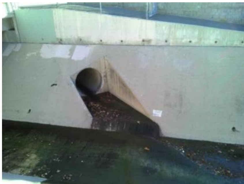
PD 1256/PD 1713 Ground-Level View
