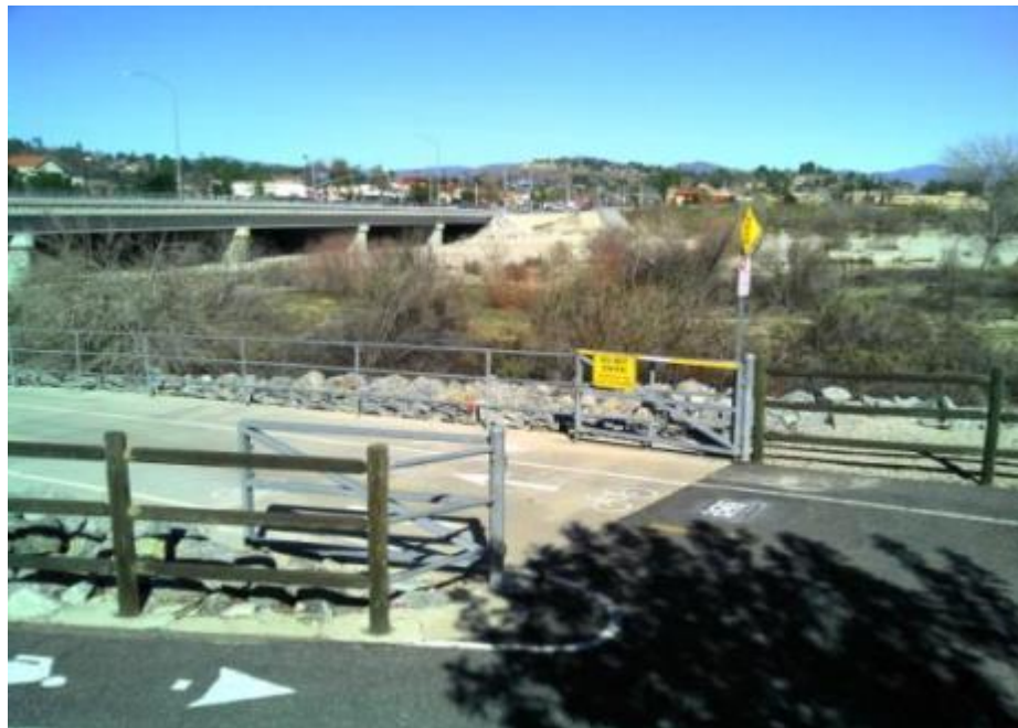
SNTCLR_7_R-A Ground-Level View
