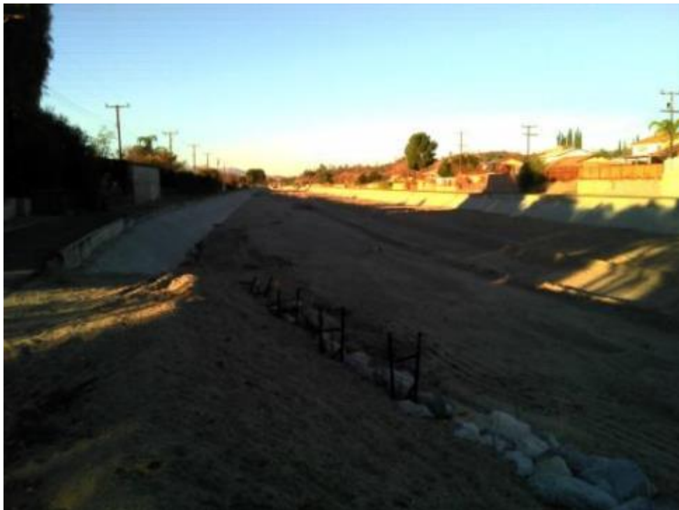
SNTCLR_BC_PARK Ground-Level View
