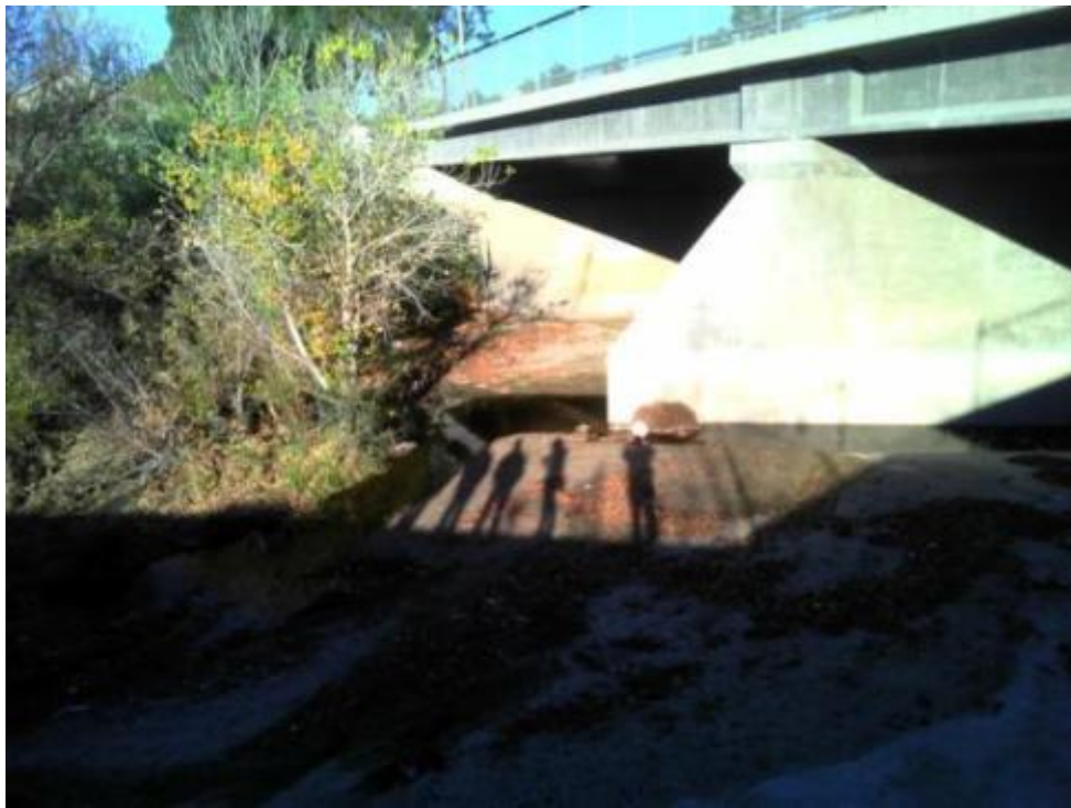
SNTCLR_BC_SWAMP Ground-Level View
