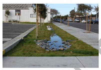
Figure 8: Vegetated swale (Signal Hill, CA).
