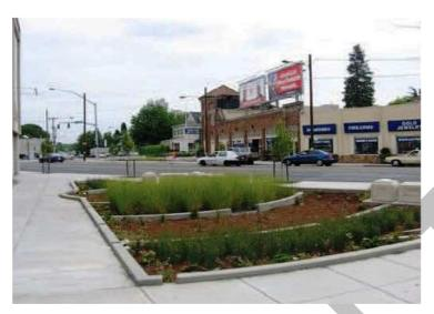
Figure 6: Bioretention system (Model for Living Streets Design Manual, 2011).
