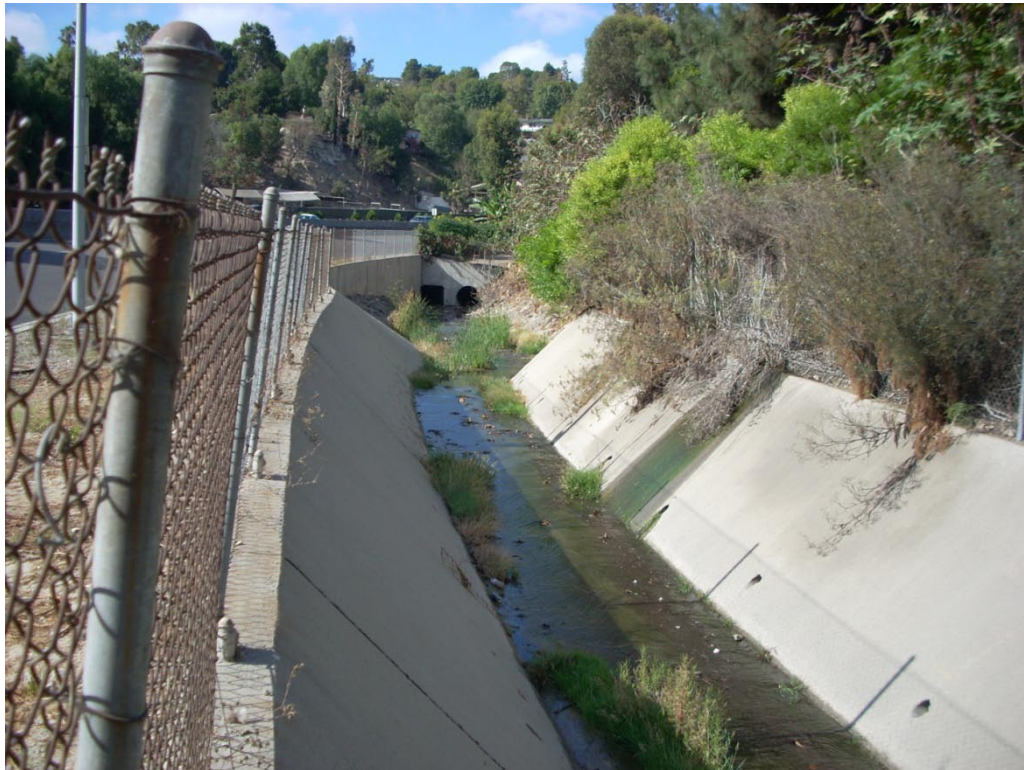
Figure 2.10 Looking South/Upstream RDD 275 along Crenshaw Boulevard
