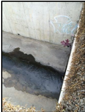
Figure 5: Outfall ID 57 with moderate flow.
