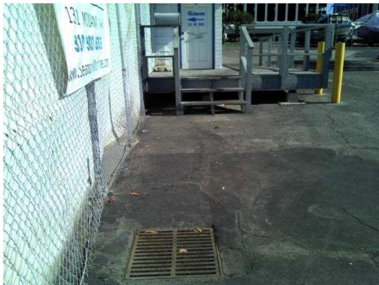
**Figure 14. Example Catch Basin at Seamark**
