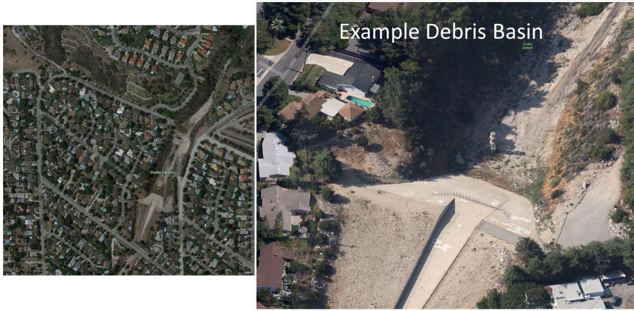
Figure 6A-1. Example debris basin. There are 162 such structures at the base of mountain canyons at the natural-urban interface. The overflow weirs are the start of the storm drain network.
