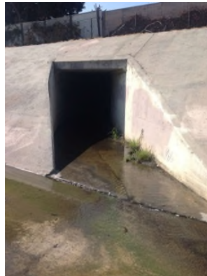
Discharge to Torrance Lateral
