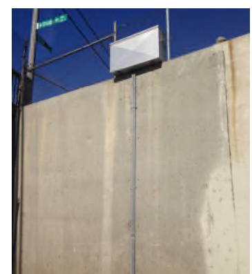
Existing Monitoring Equipment
