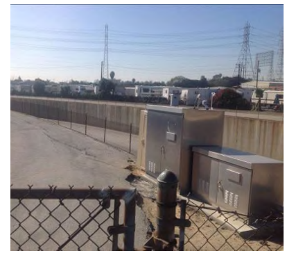
Existing Monitoring Equipment
