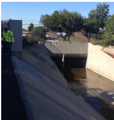
Existing Monitoring Equipment
