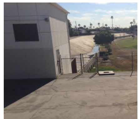
Upstream View of Avalon Pump Station
