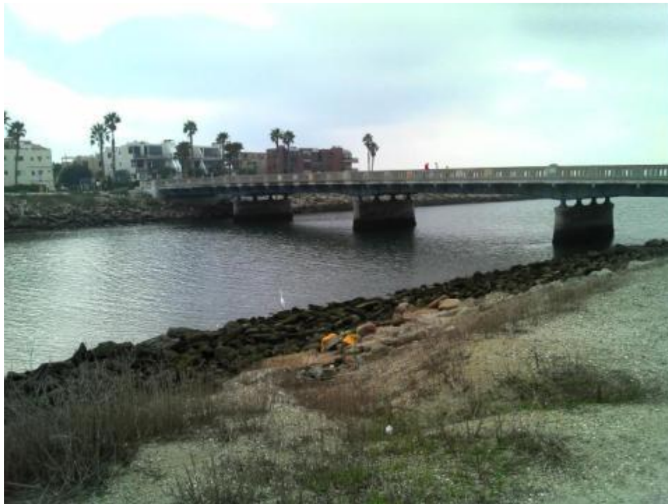
BCE_PAC Ground-Level View
