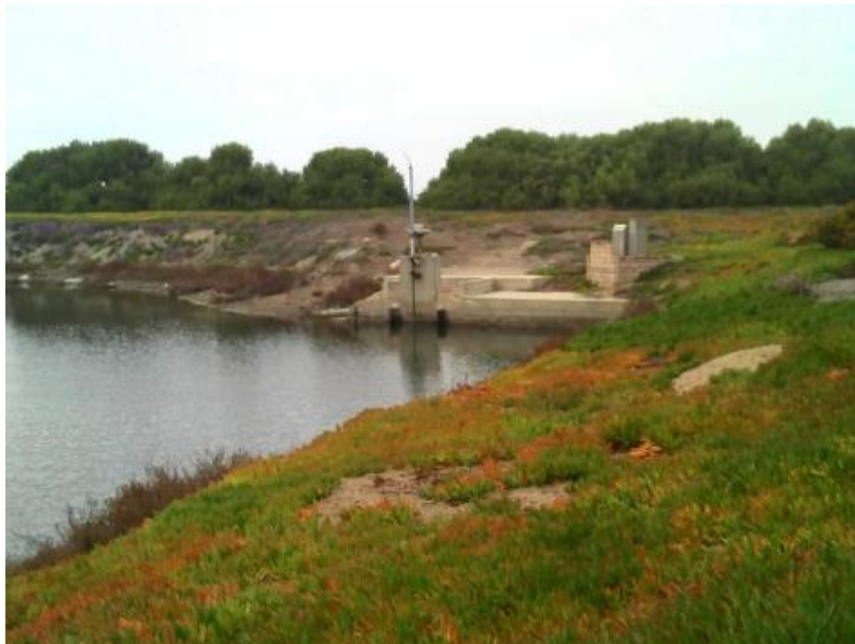
DRL_BCE Ground-Level View
