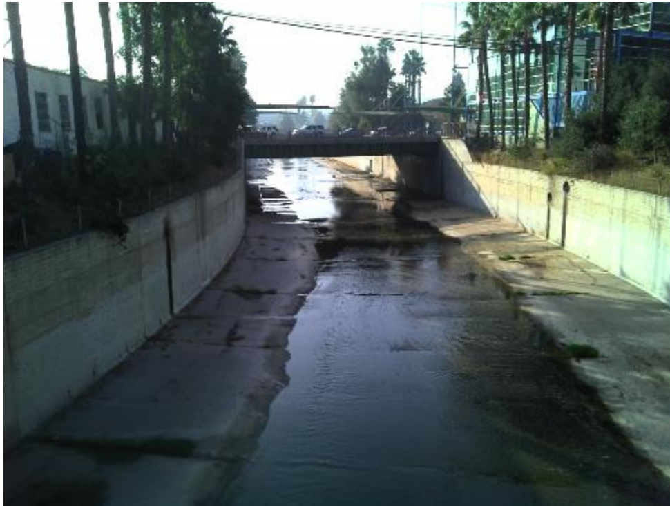
BC_01_WAS Ground-Level View
