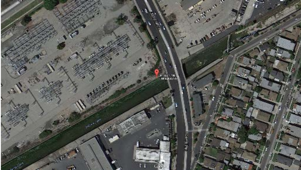
BC_SW_FAI Aerial View
