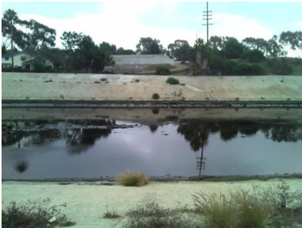
BCE_MCC Ground-Level View
