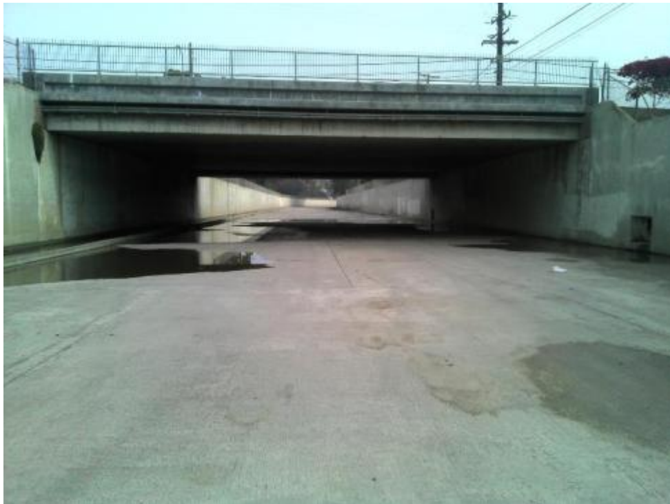
CC_CEN Ground-Level View
