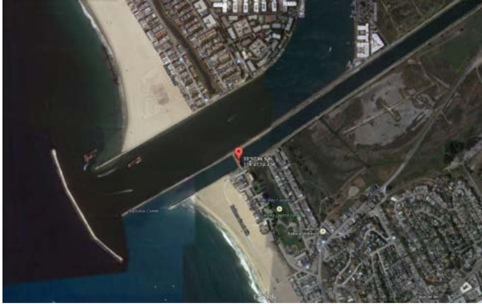
BCE_PAC Aerial View
