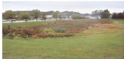
Figure 1. Example of a Dry Extended Detention Basin
