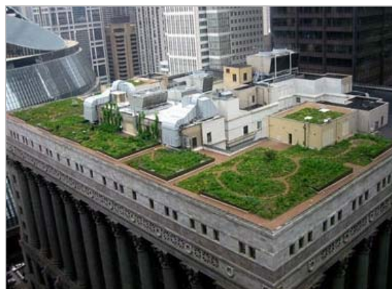
Green roof on top of Chicago City Hall. Dept. of Energy, NREL / Katrin Scholz-Barth
