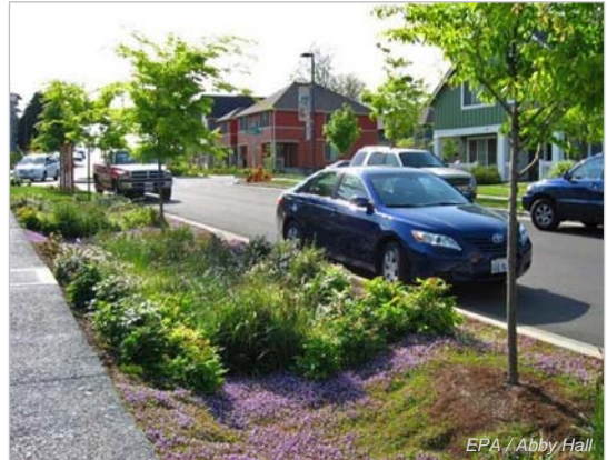
Seattle’s SEA Street (Street Edge Alternatives) project includes bioswales and permeable pavement.
