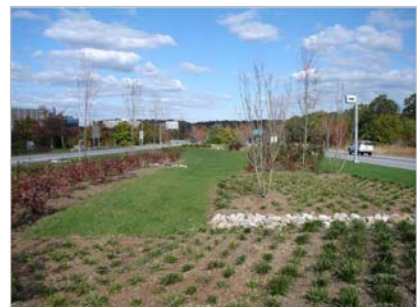
Highway divider strip before and after the retrofit of an infiltration swale.
