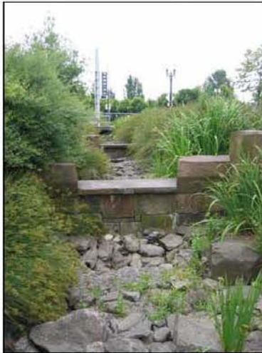
A rain garden manages runoff from impervious surfaces such as roofs and paved areas.
