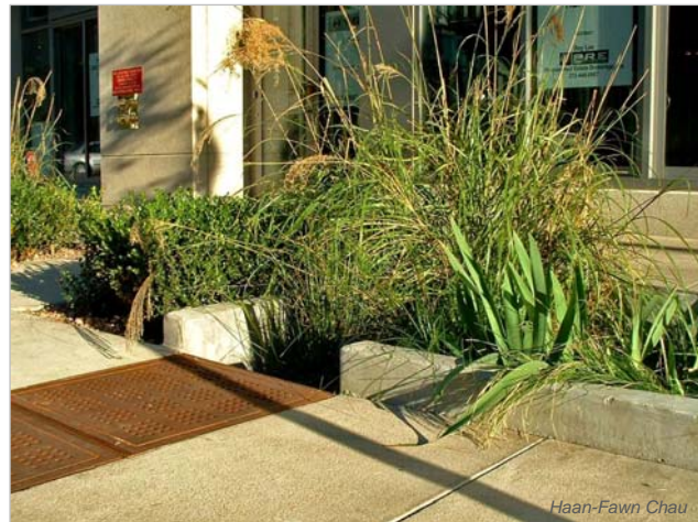
A curb cut that directs water from the street and sidewalk into a bioswale. 1100 S. Hope Street in downtown Los Angeles.
