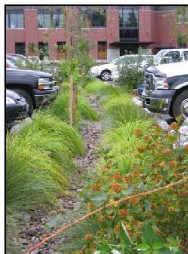
Parking lot runoff is allowed to infiltrate through a vegetated bioretention area
