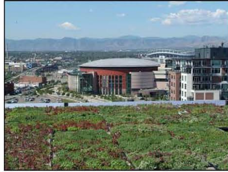
Green roofs capture rainfall, promote evapotranspiration, and offer energy savings. This is a photo of a green roof on the EPA Region 8 building in Denver, CO.
