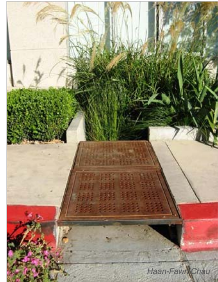
Curb cut that directs water from the street into a bioswale. Voluntarily installed at 1100 S. Hope Street in downtown L.A.
