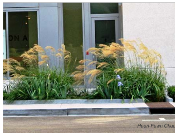
A curb cut and bioswale at 1100 S. Hope Street in downtown Los Angeles. Haan-Fawn Chau
