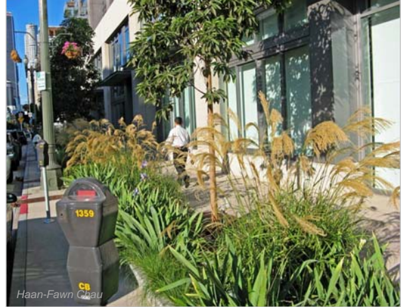
Bioswales at 1100 S. Hope Street in downtown L.A.
