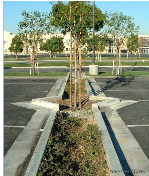
A vegetated swale with curb cuts in the parking lot of a shopping center at 8500 Firestone Blvd., Downey, CA.
