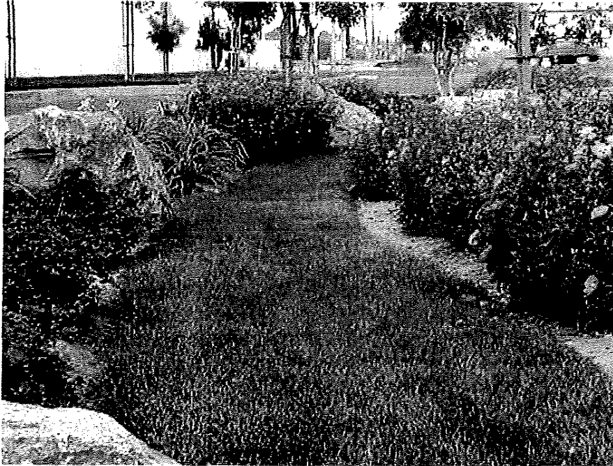
Figure 8: Vegetated Swale (Downey, CA).
