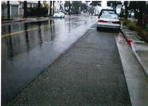
Figure 4: Permeable pavement during a storm event ( Model for Living Streets Design Manual, 2011 ).
