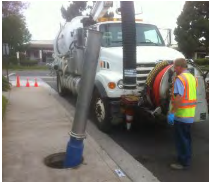
Catch Basin Cleaning Using a Vacuum Truck
