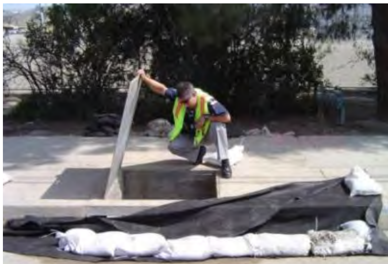
Inspection of catch basin BMPs
