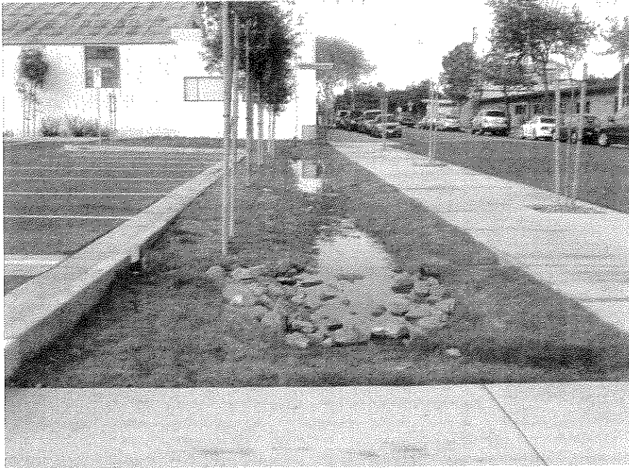
Figure 2: Vegetated Swale (Signal Hill, CA).
