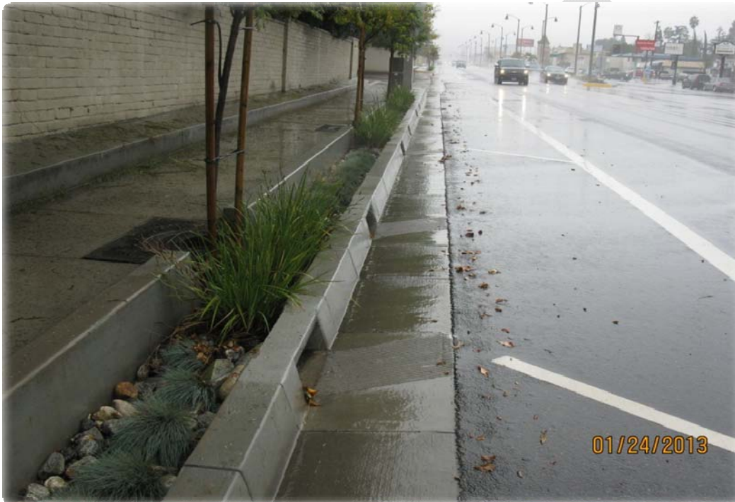
Figure 8: Vegetated swale. Courtesy, Photo courtesy of Los Angeles County, Rosemead Boulevard.
