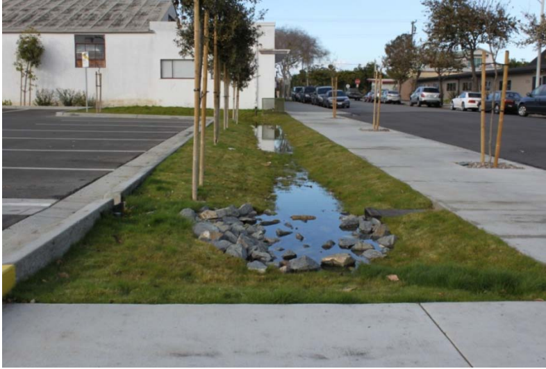
Figure 8: Vegetated swale (Signal hill, CA).
