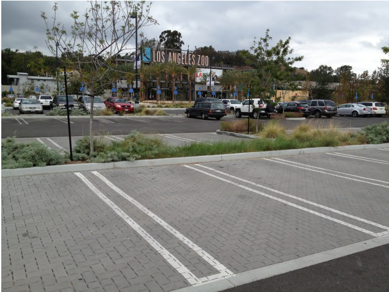
Porous pavement parking stalls and bioretention at the Los Angeles Zoo (Photo credit: Tetra Tech)
