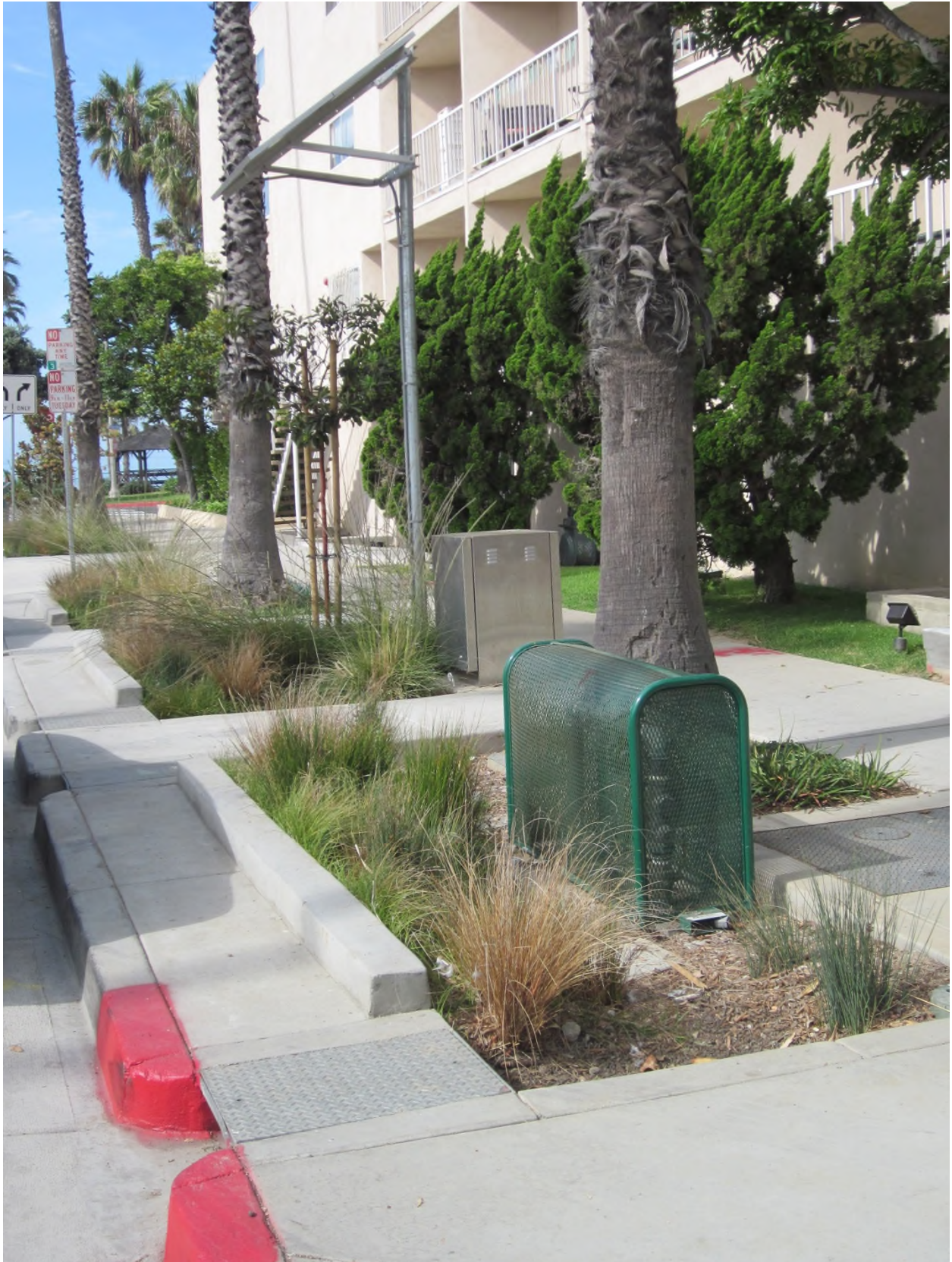
Bioretention sidewalk retrofits in Santa Monica, CA
