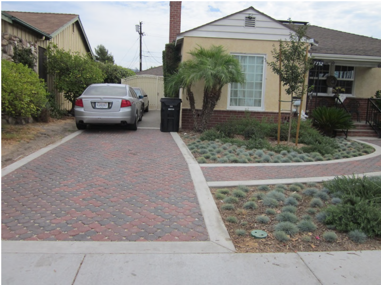
Porous pavement and xeriscape in Los Angeles, CA
