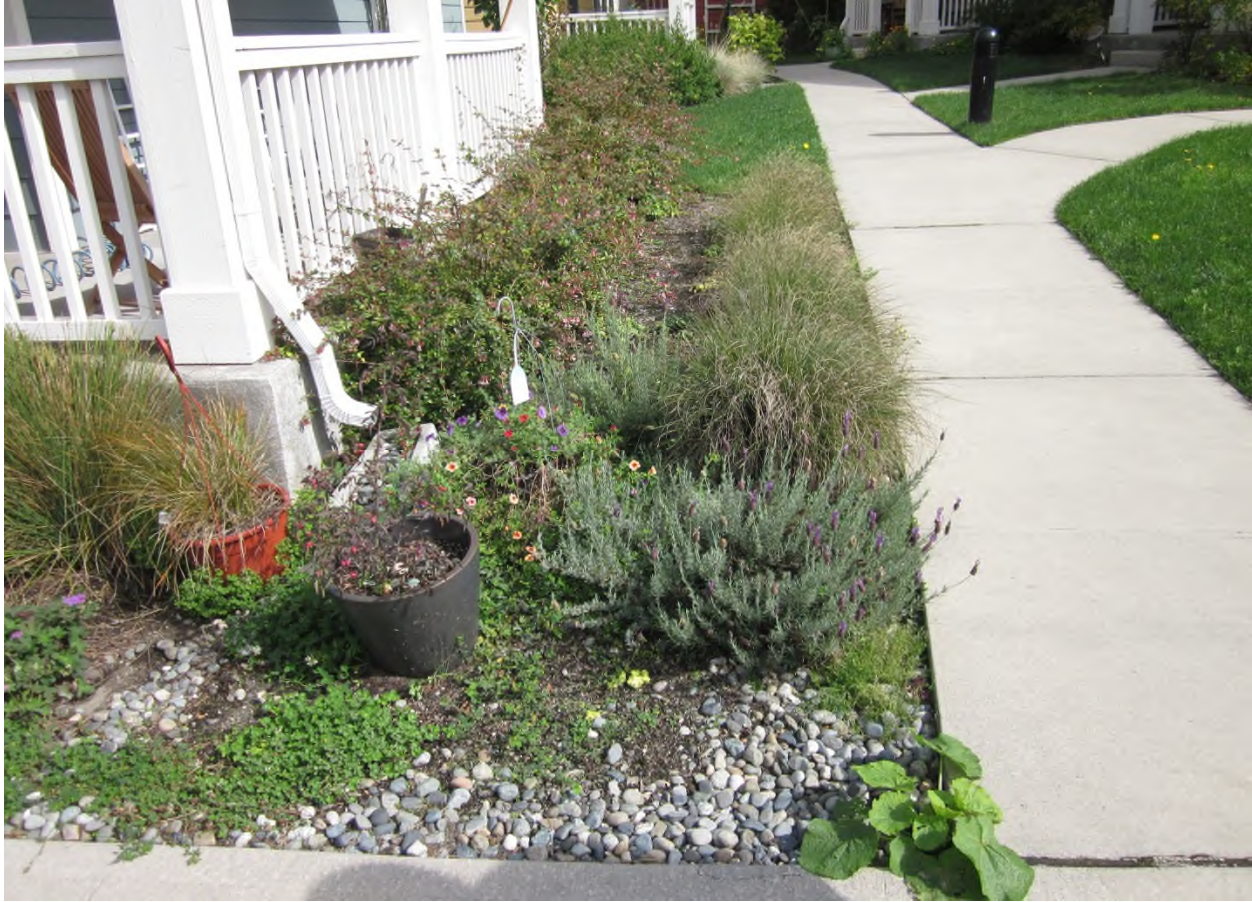
Residential downspout disconnection in Seattle, WA
