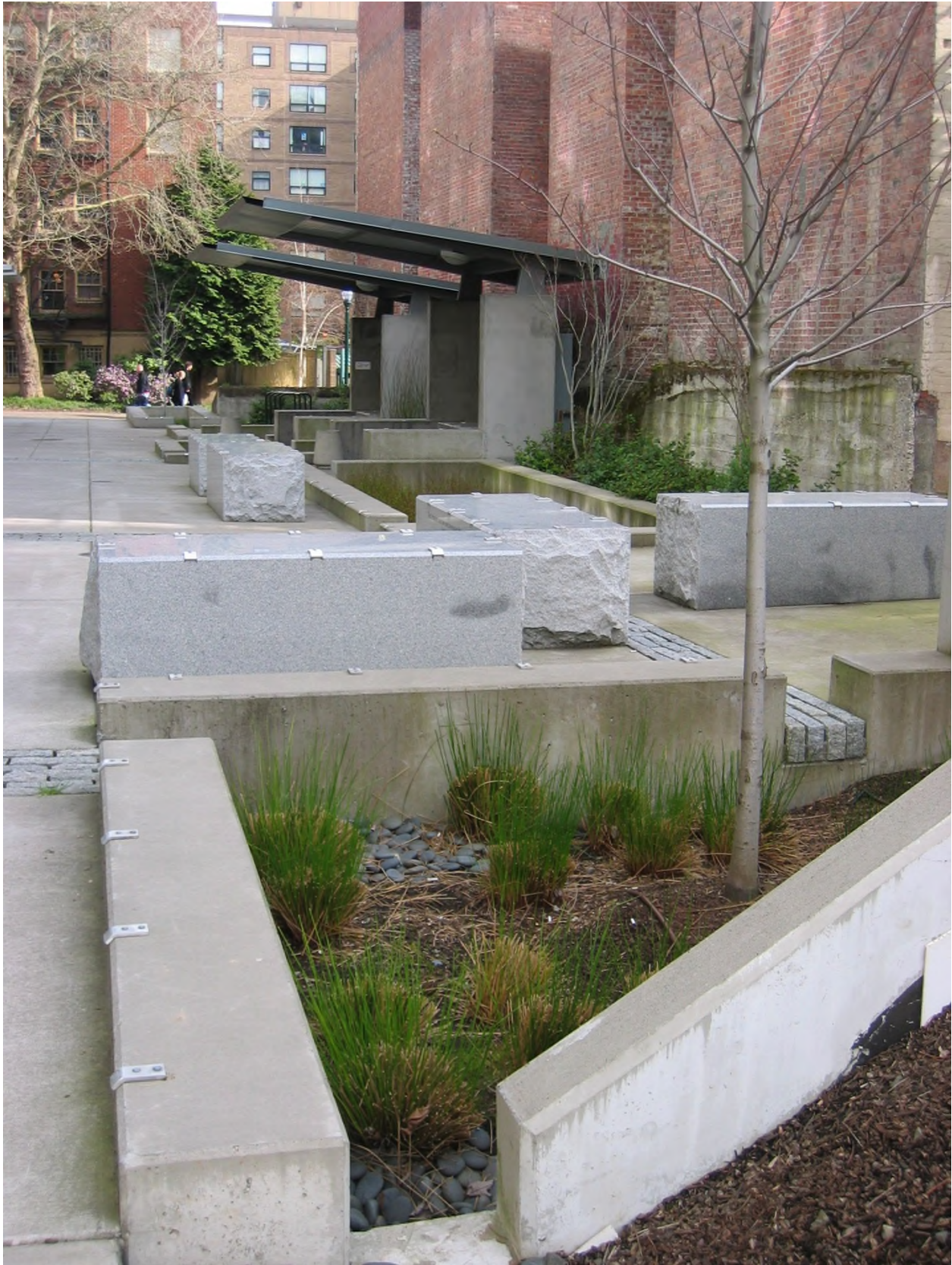
Bioretention in a plaza gathering space in Portland, OR (Photo credit: M. Frey)
