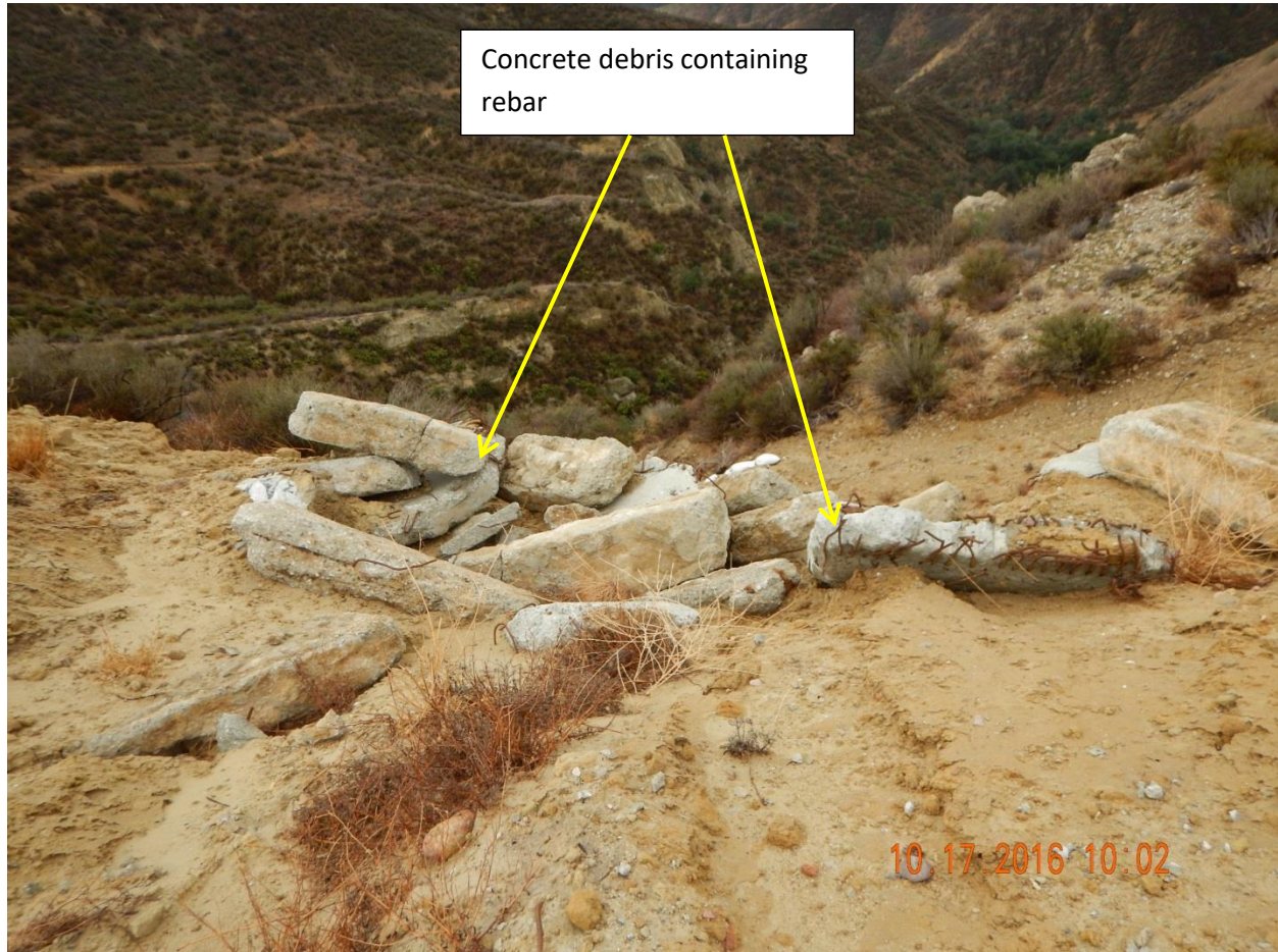
Photo 11. This photo shows concrete debris partially buried in Parcel 2821-002-025 from sediment build up. The pieces of concrete debris contained rebar. This photo was taken near latitude: 34 18.574 and longitude: -118 37.078.
