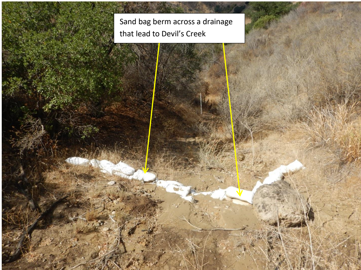
Photo 9. This photo shows a sand bag berm located in drainage that leads to Devil's Creek. This photo was taken on parcel 2821-002-025, at latitude: 34 18.568 and longitude: -118 37.358. This area lacked erosion control best management practices, and there was loose sediment accumulated behind the berm.
