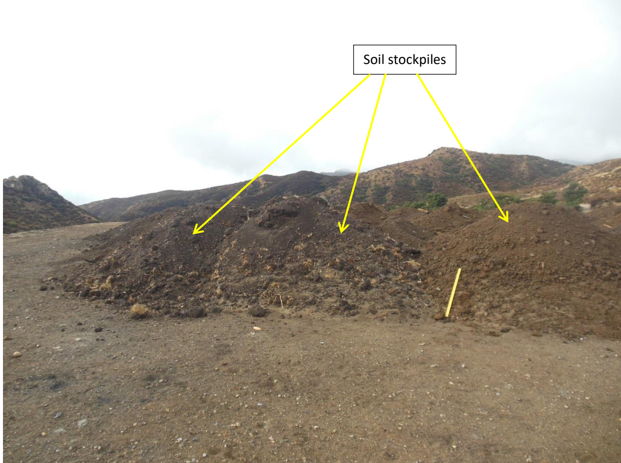
Photo 28. This photo shows stockpiles of soil found in Parcel 2821-009-031. This area lacked erosion or sediment control BMPs. This photo was taken near latitude: 34 18.264 and longitude -118 36.644.
