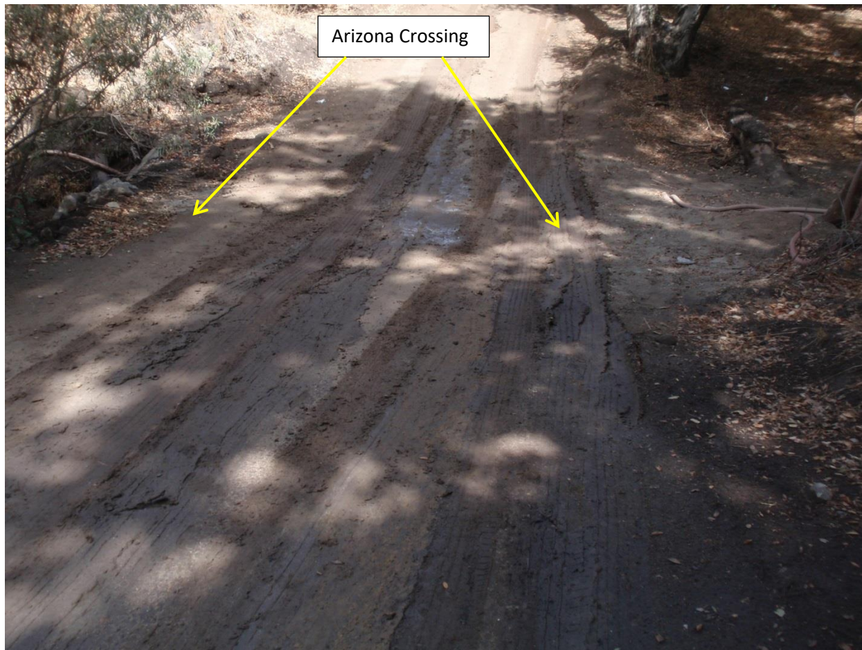
Photo 32. This photo shows an Arizona crossing in Ybarra Creek in Parcel 2821-009-023. This photo was taken near latitude: 34 18.158 and longitude:-118 36.665.
