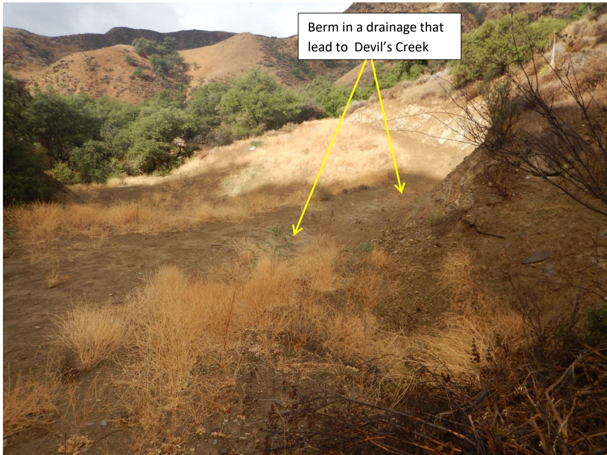
Photo 3. This photo shows another view of the berm in drainage that lead to Devil's Creek that was also shown in Photo 2. This photo was taken in Parcel 2821-002-025 at latitude: 34 18.729 and longitude: -118 37.367.
