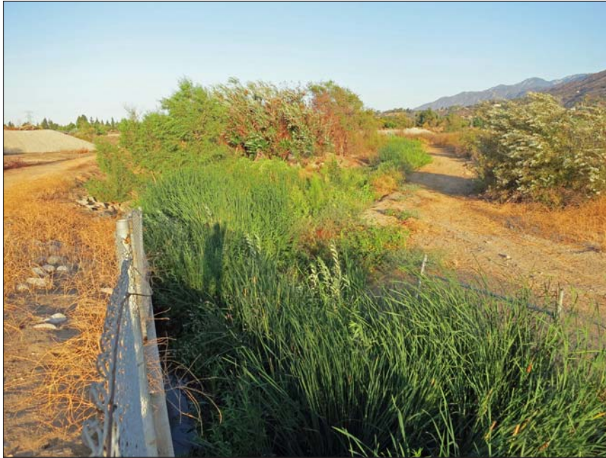
August 26, 2013. View of Beatty Channel Outlet - Reach 39.
