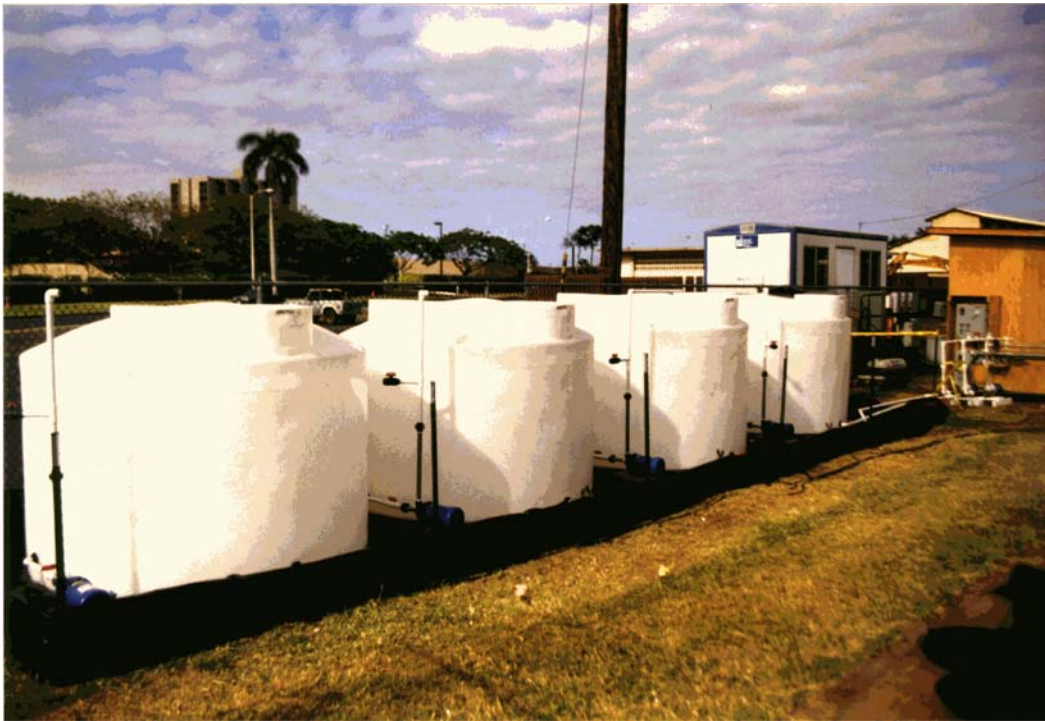
Figure 3-1. HDPE Storage Tanks Used for Blending Electrolyte Solutions
