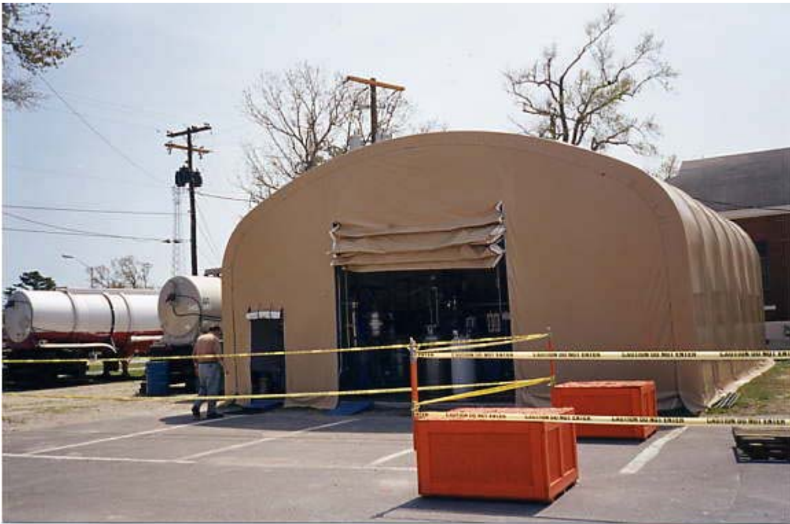
Figure 3-3. Temporary Tented Wastewater Treatment Facility
